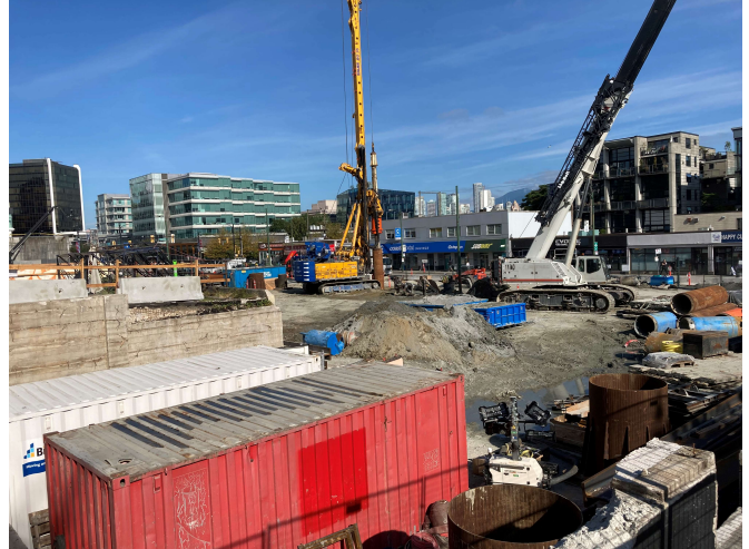
Broadway City Hall Station: Progressing with the installation of piles
