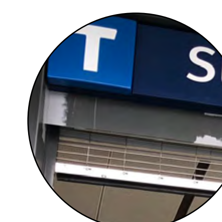
Station entrance coiling grille
