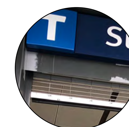
Station entrance coiling grille
