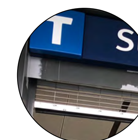
Station entrance coiling grille
