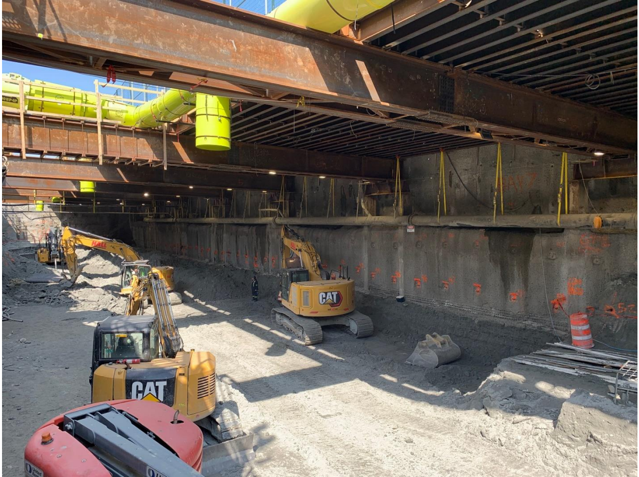
Figure 3: Mount Pleasant Station: Progressing with the excavation and shoring of the station box and headhouse.
