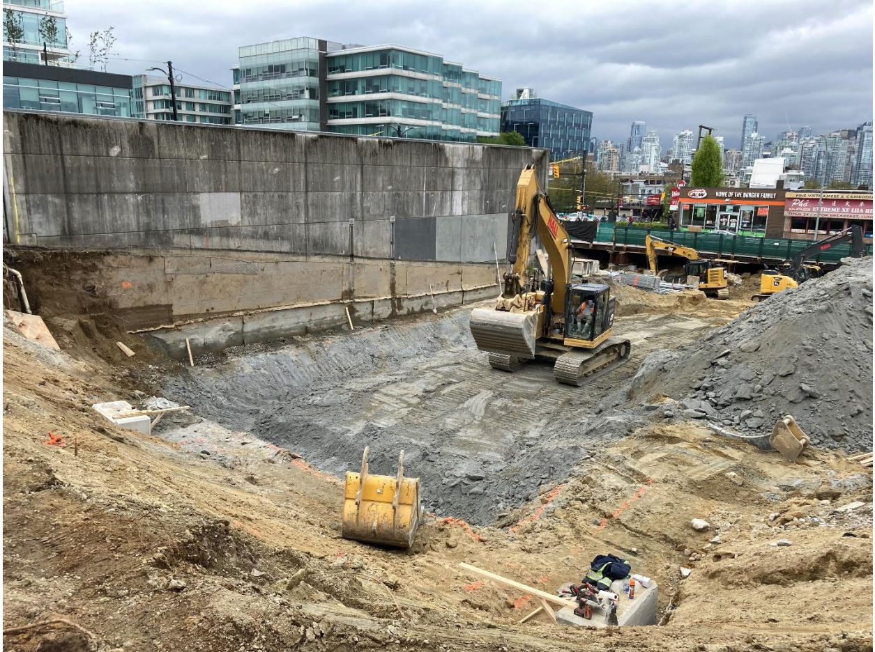
Figure 4: Broadway City Hall Station: Excavation for the headhouse begins.
