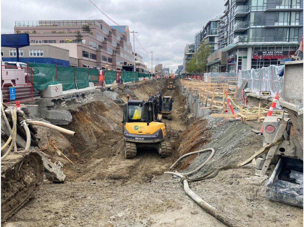
Figure 7: Arbutus Station: Progressing with the shallow excavation for the traffic deck.
