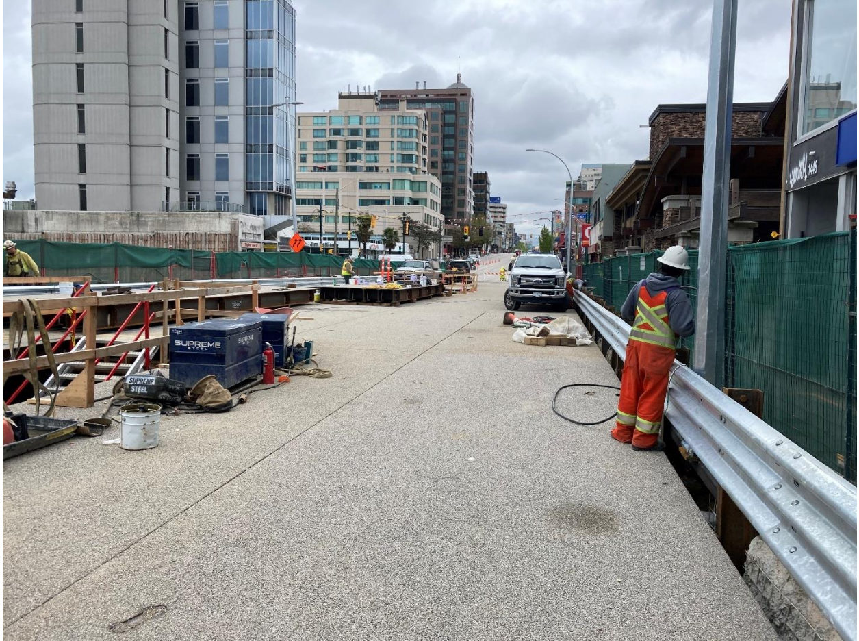
Figure 6: South Granville Station: Installation of the traffic decking from Hemlock St to Granville St.
