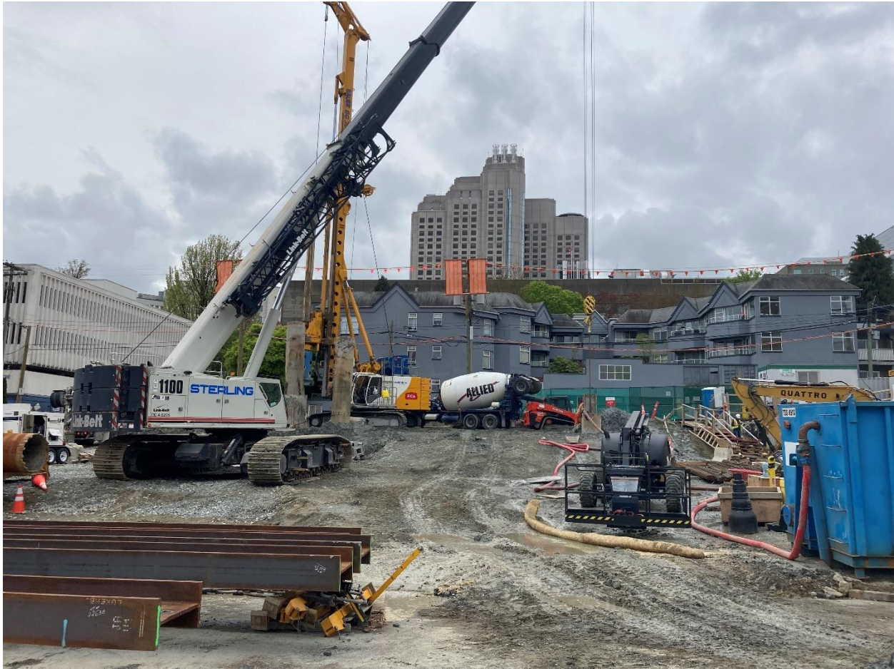
Figure 5: Oak VGH Station: Initial start of piling for the headhouse.
