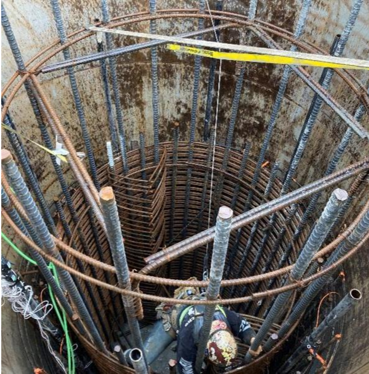
Figure 1: Elevated Guideway: Progressing with the installation of caissons for the columns.
