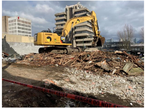
Oak VGH Station March 30, 2021. Progressing with demolition work.
