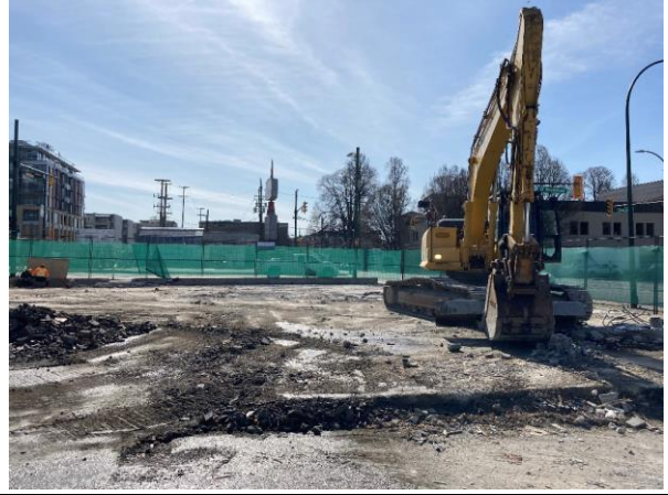
Arbutus Station March 11, 2021. Progressing with demolition work.
