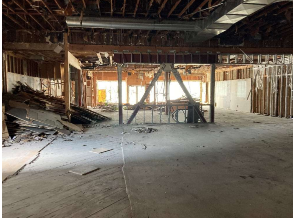
South Granville Station, April 2021. Progressing with non-structural demolition.
