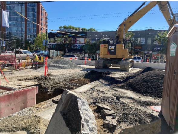
Main and 8th Utility Relocation Work: Excavating and back filling along 8th Avenue
