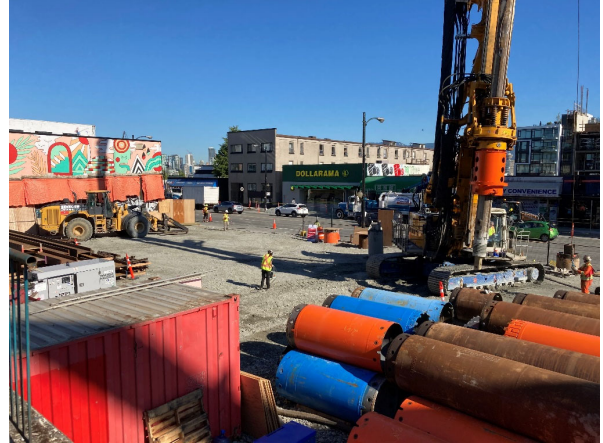
Mount Pleasant Station: Installation of columns (piles)
