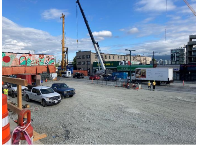
Mount Pleasant Station: Progressing with the installation of piles
