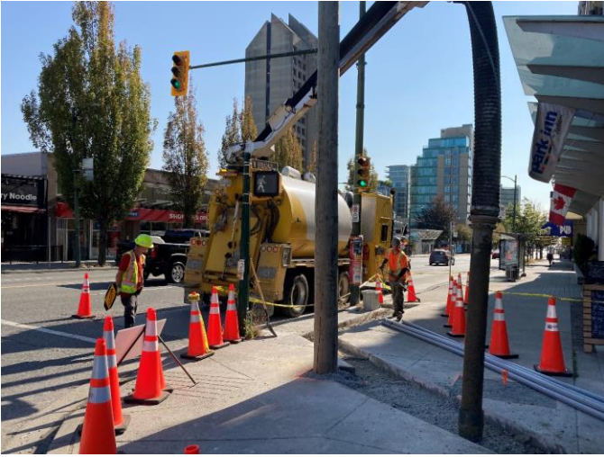
Oak-VGH Station: Hydrovac work to relocate utilities for construction
