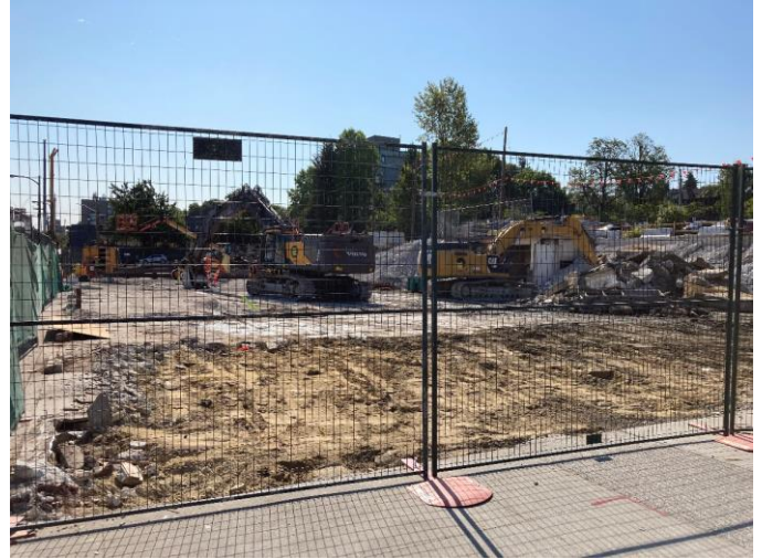
Broadway City Hall Station: Completion of demolition activities
