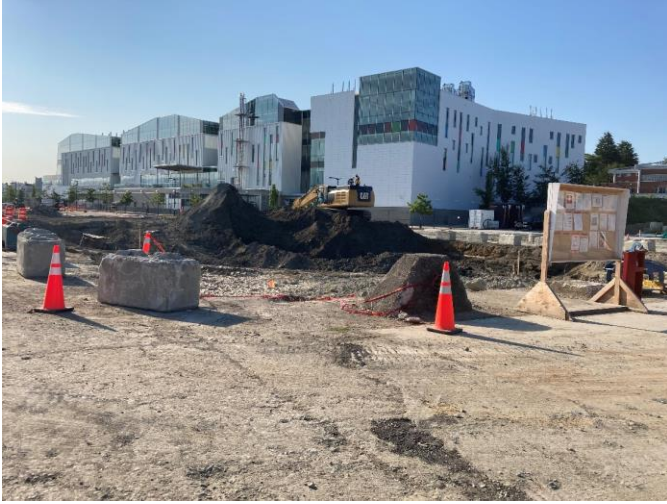
Great Northern Way-Emily Carr Station: Progressing with site excavation work
