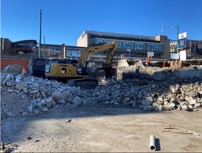
South Granville Station: Sorting of demolition debris with an excavator
