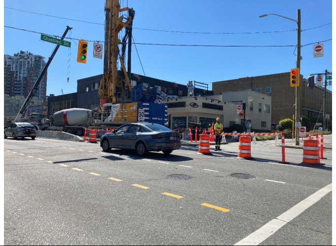
Mount Pleasant Station: Installation of piles in front of the businesses along W. Broadway, near Quebec St
