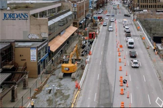
Arbutus Station: Progressing with the relocation of utilities and installation of a temporary water pipe
