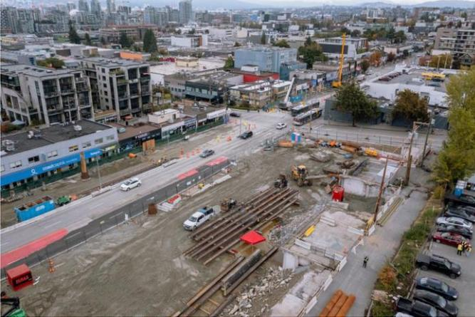
Oak VGH Station: Progressing with the installation of piles for traffic decking
