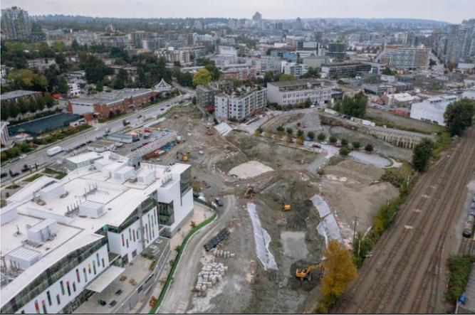
Mount Pleasant Station: Progressing with shallow excavation for decking install
