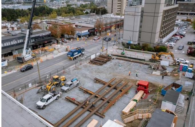
South Granville Station: Progressing with the relocation of utilities and the installation of piles for traffic decking
