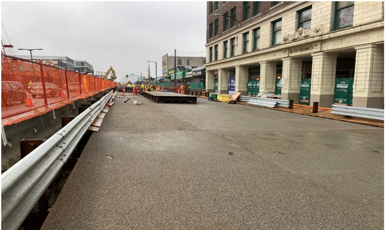
Figure 2: Mount Pleasant Station: Progressing with the installation of traffic decking.
