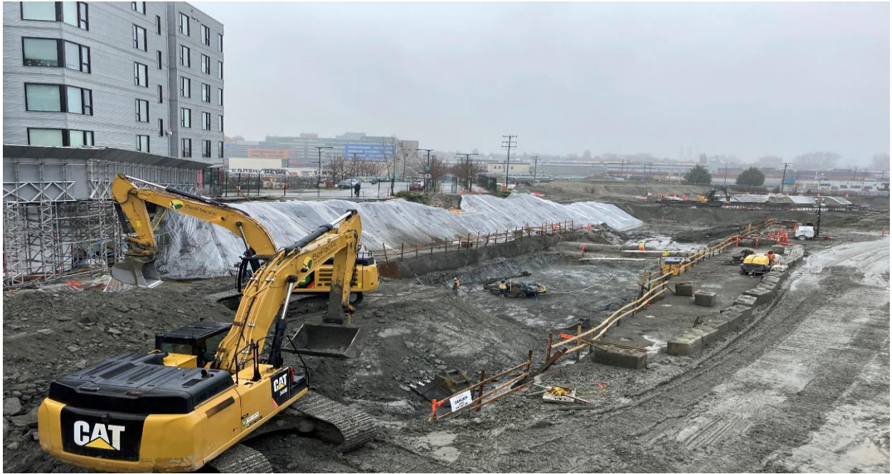
Figure 1: Great Northern Way-Emily Carr Station: Progressing with excavation, installation of wall anchors and piles.
