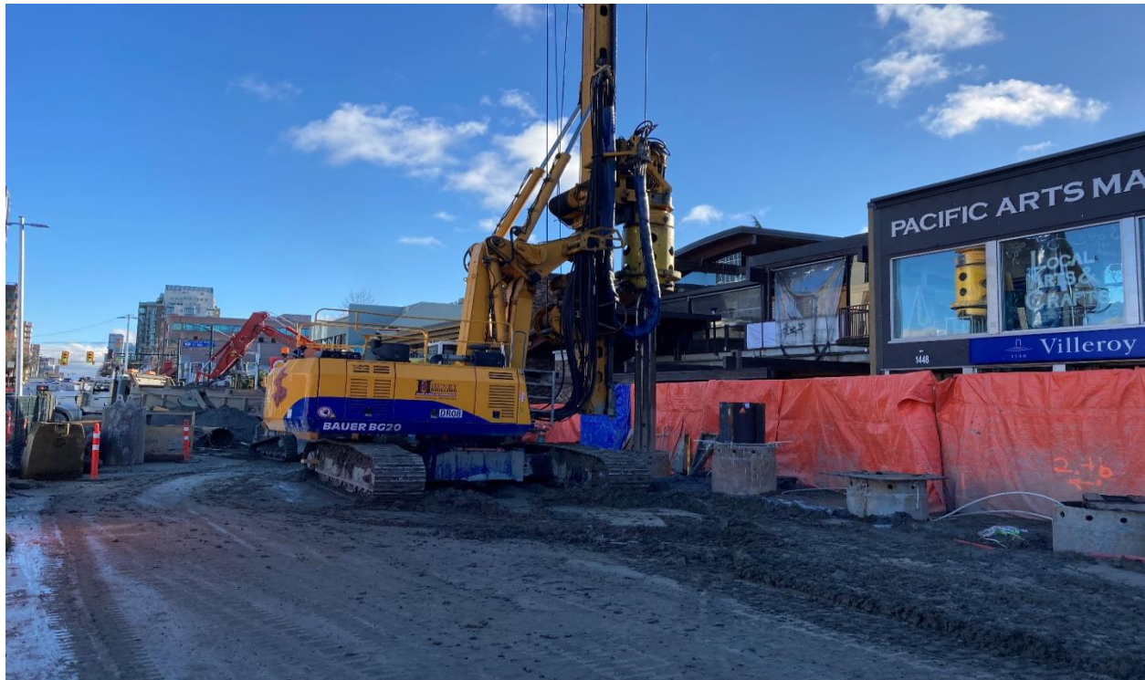
Figure 5: South Granville Station: Progressing with the installation of piles for the traffic decking.
