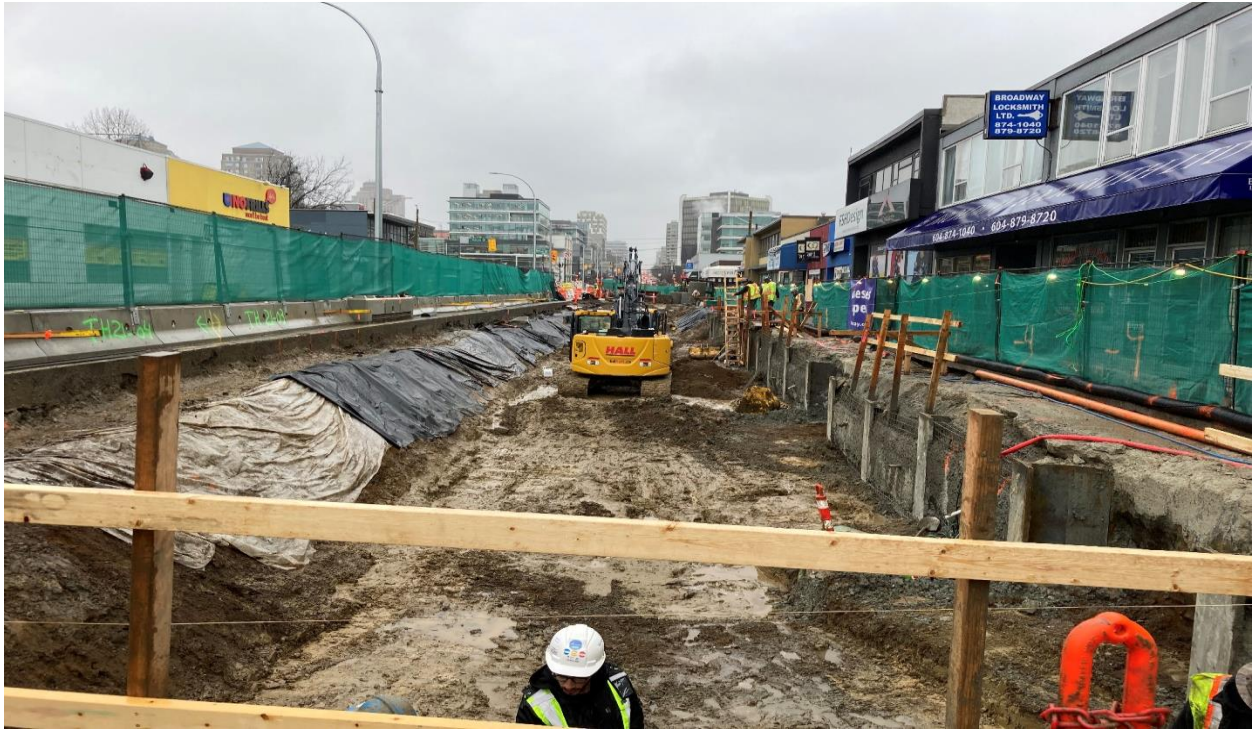
Figure 3: Broadway City Hall Station: Progressing with the excavation of the station box.
