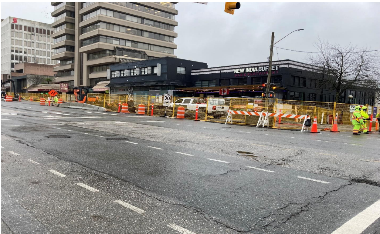
Figure 4: Oak VGH Station: Progressing with the relocation of underground utilities and installation of temporary utilities.
