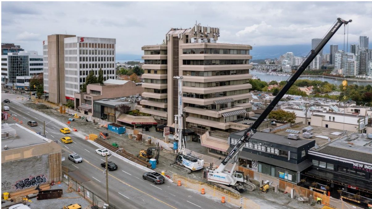
Figure 4: Oak VGH Station: Installation of piles for traffic decking
