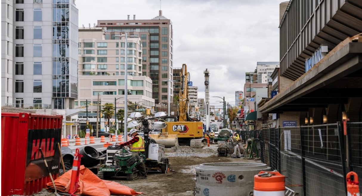
Figure 5: South Granville Station: Relocation of utilities and the installation of piles for traffic decking
