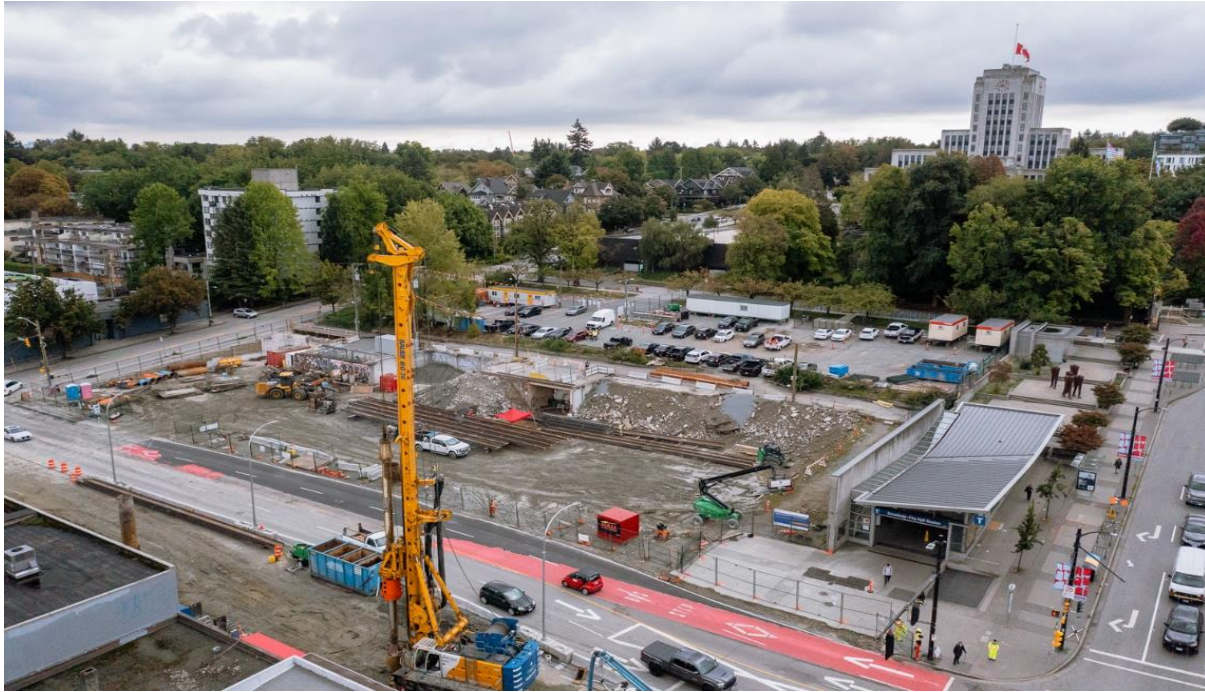
Figure 3: Broadway City Hall Station: Installation of piles for traffic decking
