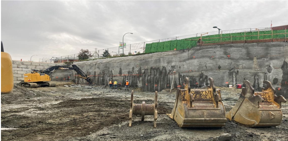
Figure 1: Great Northern Way-Emily Carr Station: Excavating the transition to the face of the portal tunnel
