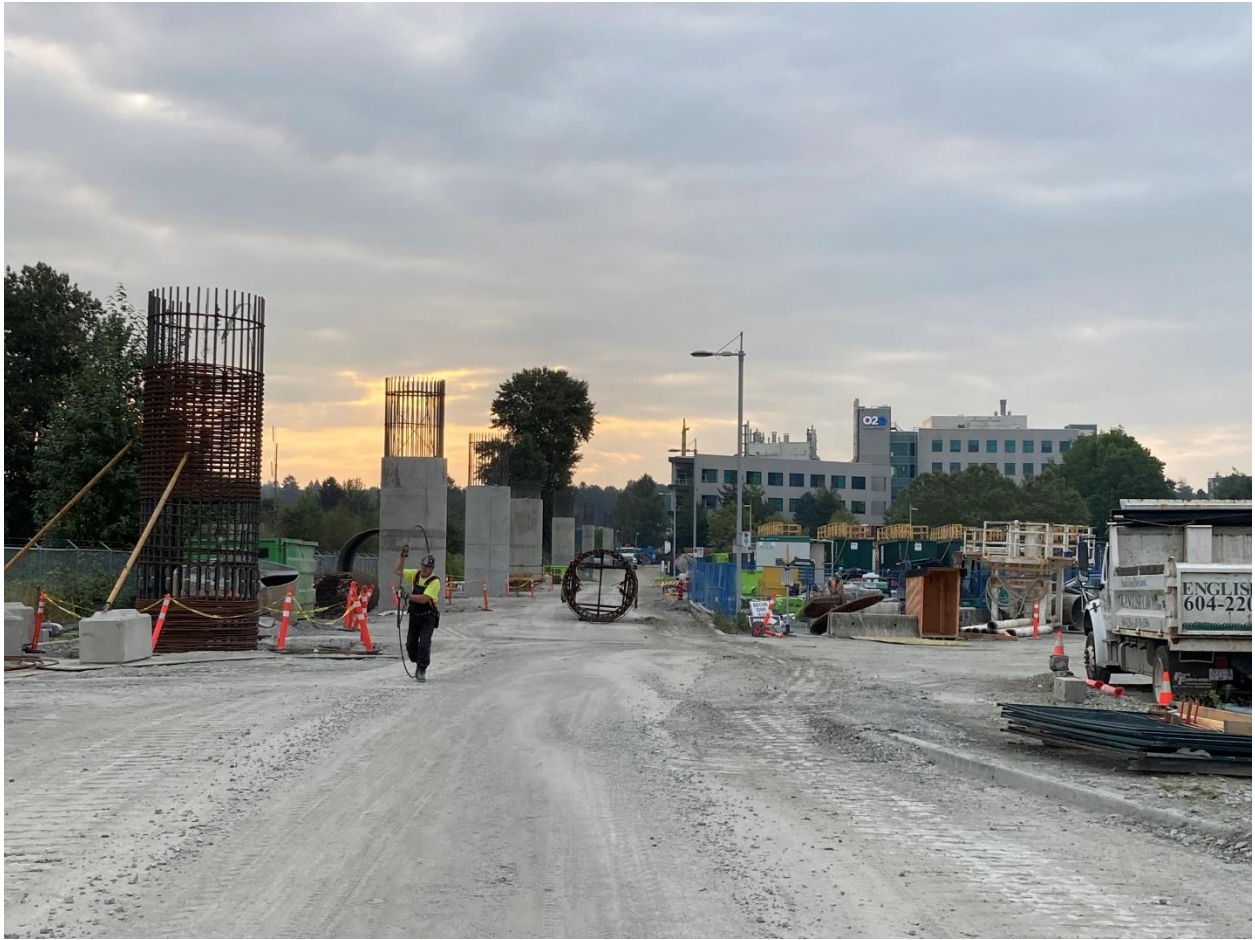
Figure 1: Elevated Guideway: Progressing with the installation of columns for the elevated guideway.
