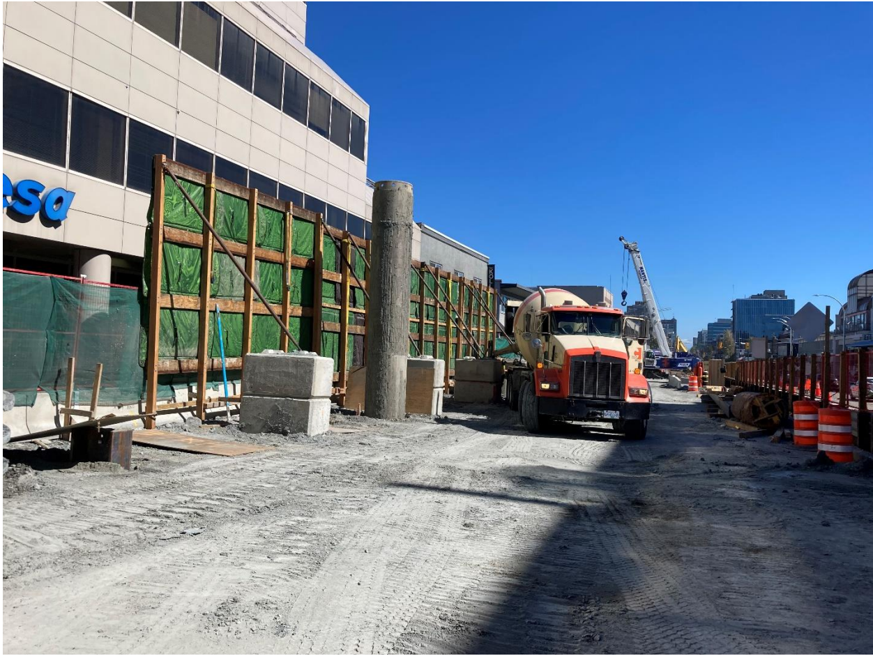
Figure 7: Arbutus Station: Progressing with the installation of piles along the north side of W. Broadway to support the traffic decking.
