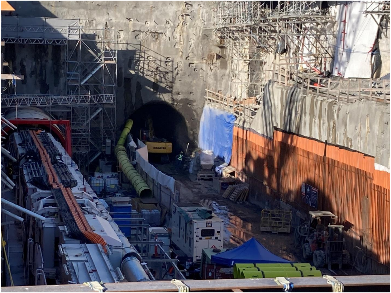
Figure 2: Great Northern Way-Emily Carr Station: Progressing with the mined tunnel excavation and shoring.
