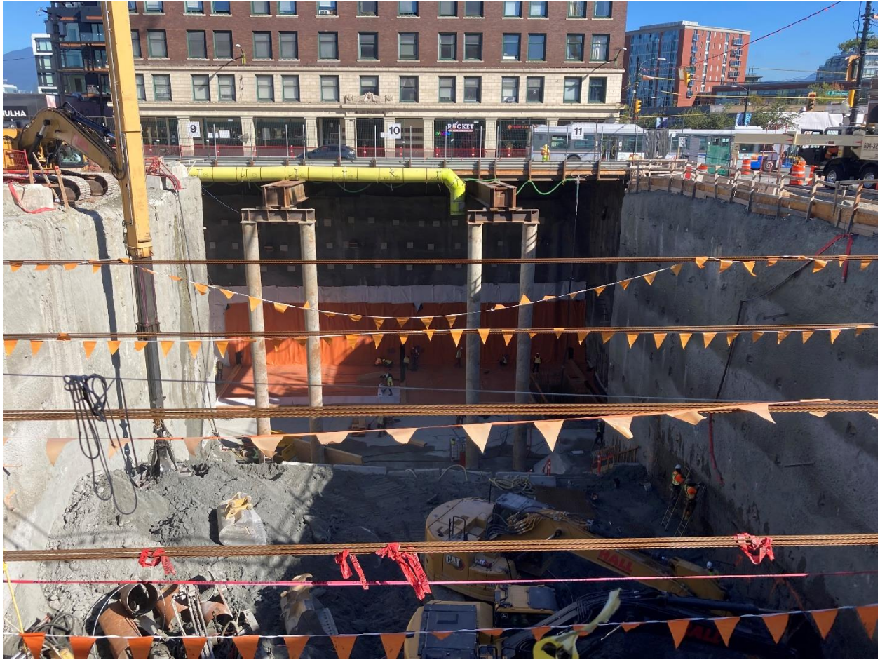
Figure 3: Mount Pleasant Station: Progressing with the excavation and shoring of the headhouse excavation and the waterproofing within the station box.
