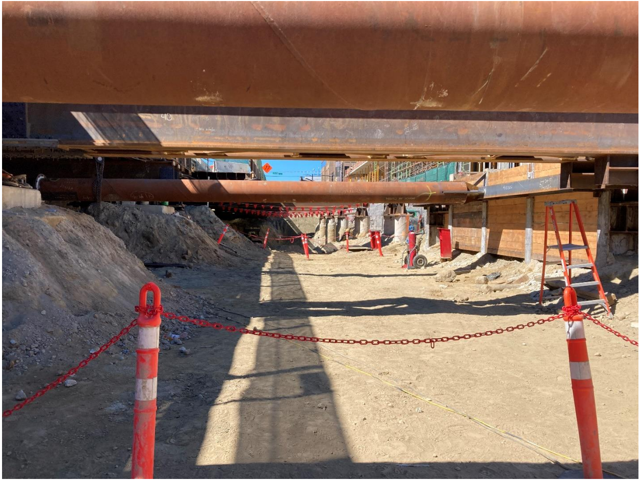
Figure 6: South Granville Station: Progressing with the installation of support girders and struts to support the station box excavation.
