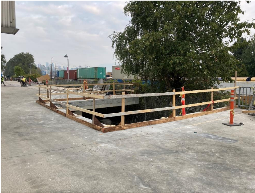
Figure 1: Elevated Guideway: Progressing with the sectional removal of a parkade slab for the installation of columns that will support the elevated guideway.
