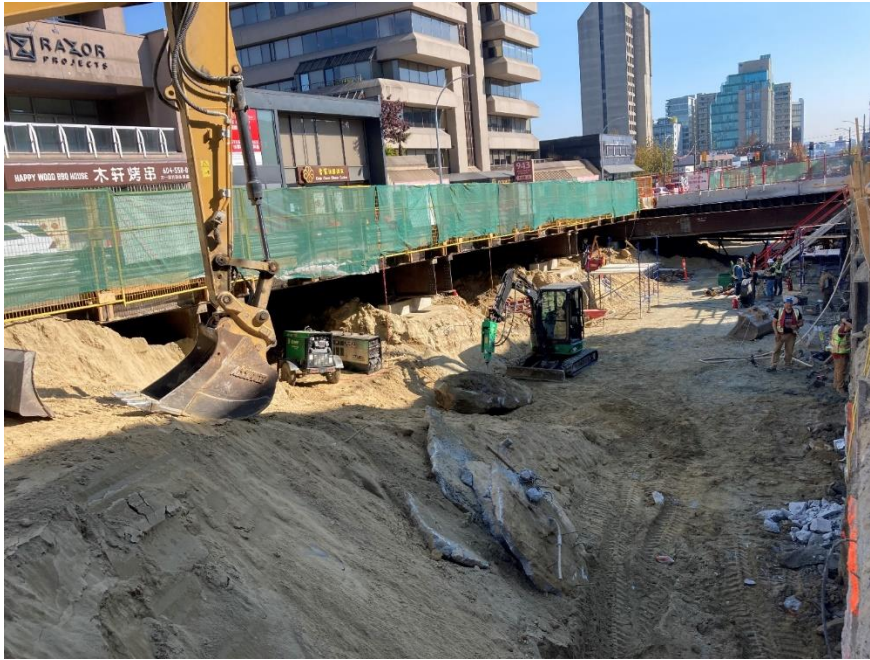
Figure 5: Oak VGH Station: Progressing with the installation of the supporting girders, struts, and traffic decking.
