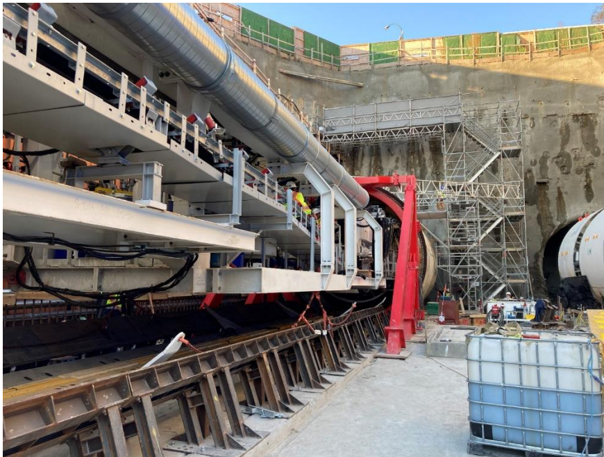
Figure 2: Great Northern Way-Emily Carr Station: Progressing with preparations to launch the first TBM.
