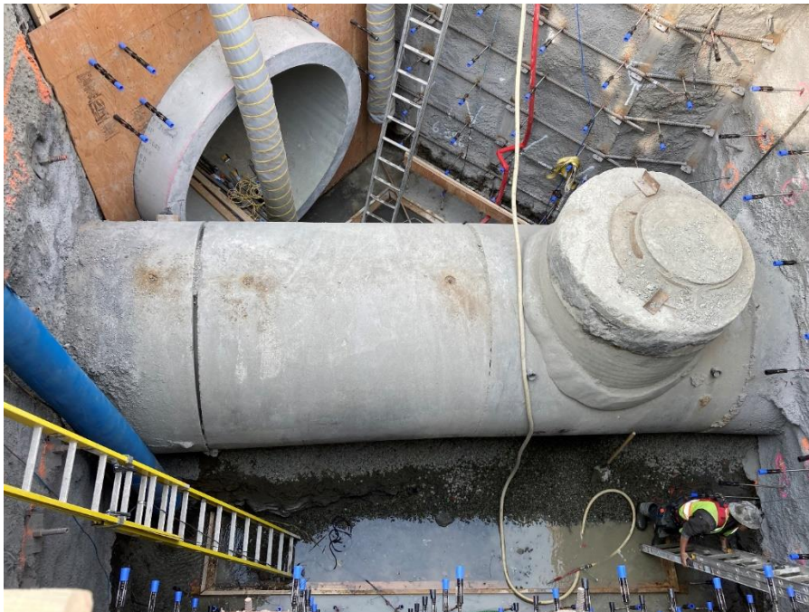
Figure 4: Broadway City Hall Station: Progressing with the re-routing and tie-in of the Cambie combined storm and sewer utility.
