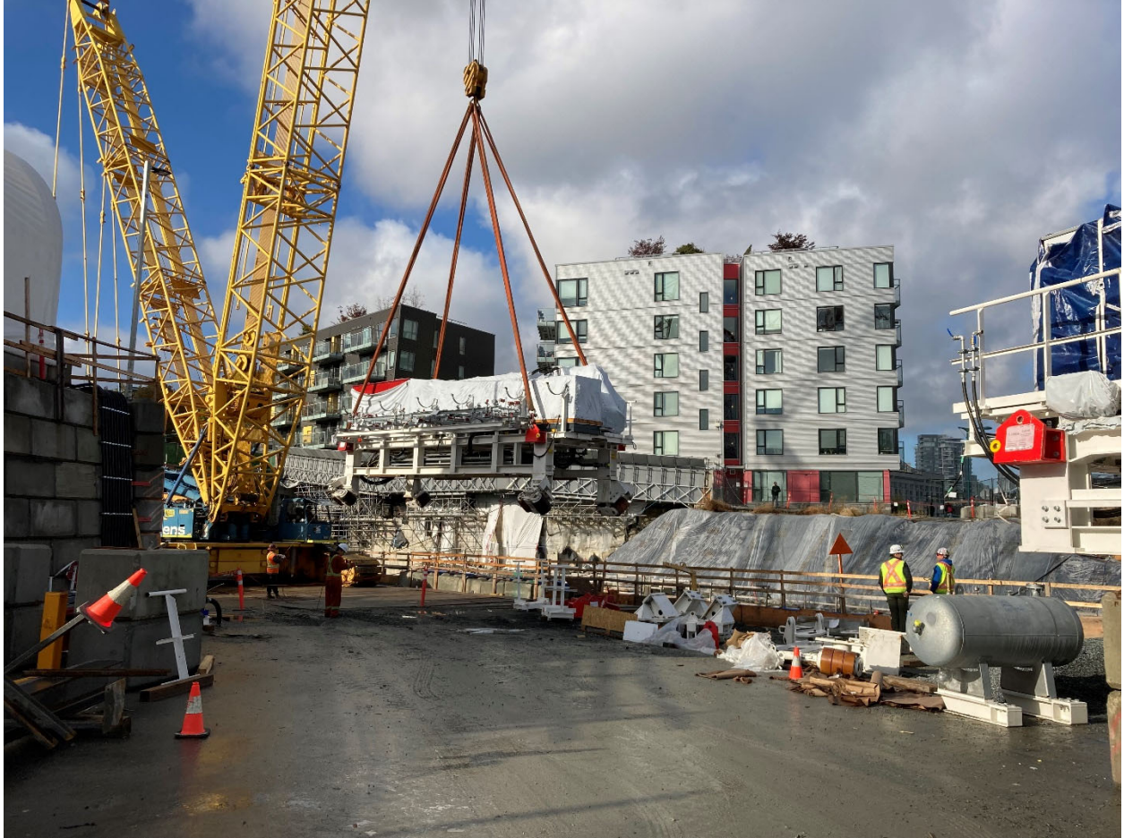
Figure 2: Great Northern Way-Emily Carr Station: Progressing with the assembly of the second Tunnel Boring Machine.
