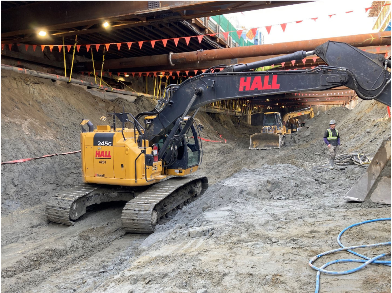
Figure 6: South Granville Station: Progressing with the excavation and shoring of the station box.
