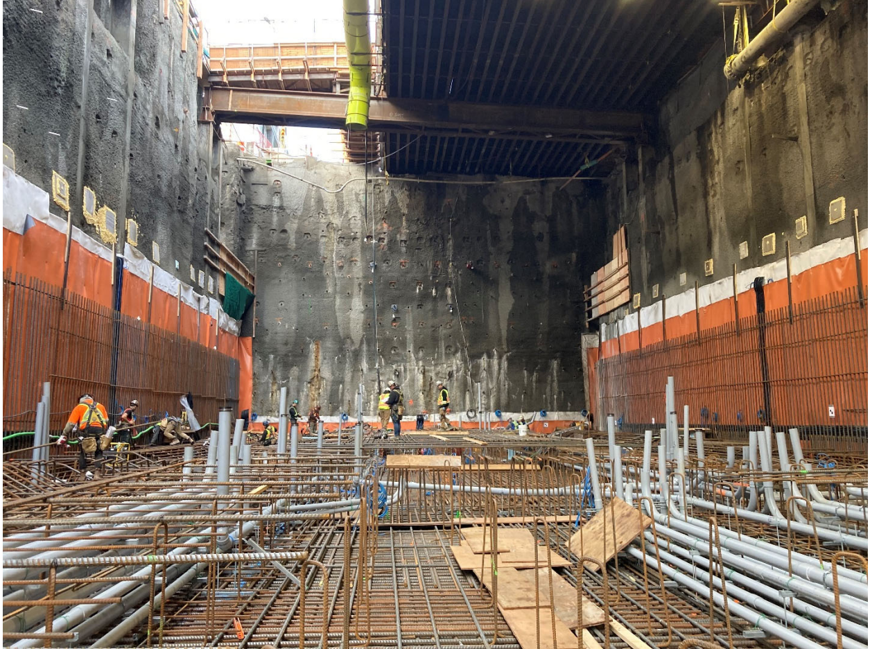
Figure 3: Mount Pleasant Station: Progressing with the installation of waterproofing, rebar and conduit within the station box excavation.
