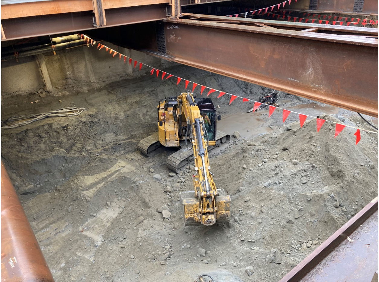
Figure 5: Oak-VGH Station: Progressing with the excavation and shoring of the station box.
