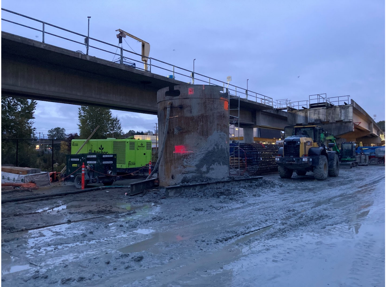
Figure 1: Elevated Guideway: Progressing with the installation of caissons for the elevated guideway.
