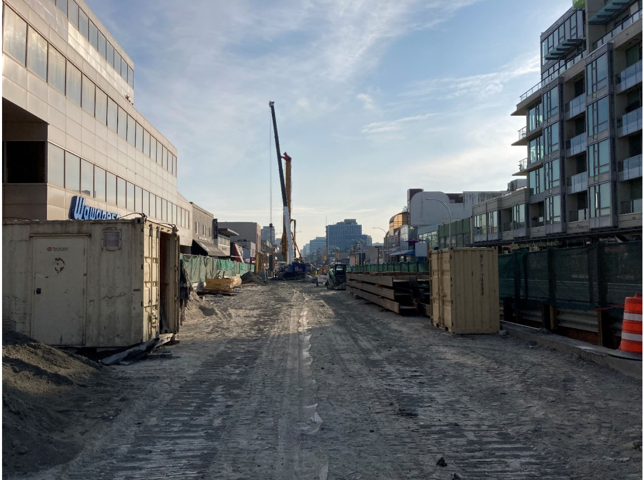
Figure 7: Arbutus Station: Progressing with the installation of piles to support the traffic decking.
