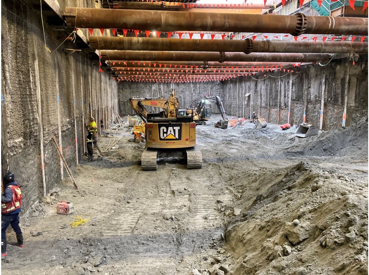
Figure 4: Broadway-City Hall Station: Progressing with the excavation and shoring of the station box.
