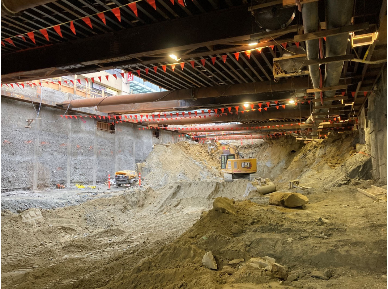
Figure 5: Oak-VGH Station: Progressing with the bulk excavation of the station box.
