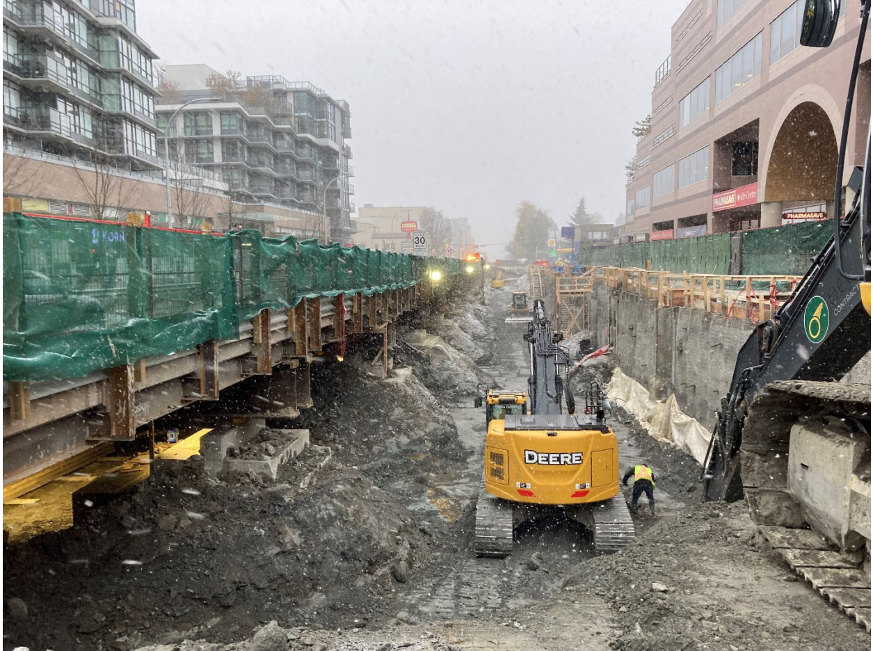
Figure 7: Arbutus Station: Progressing with shallow excavation in anticipation of the placement of the traffic deck.
