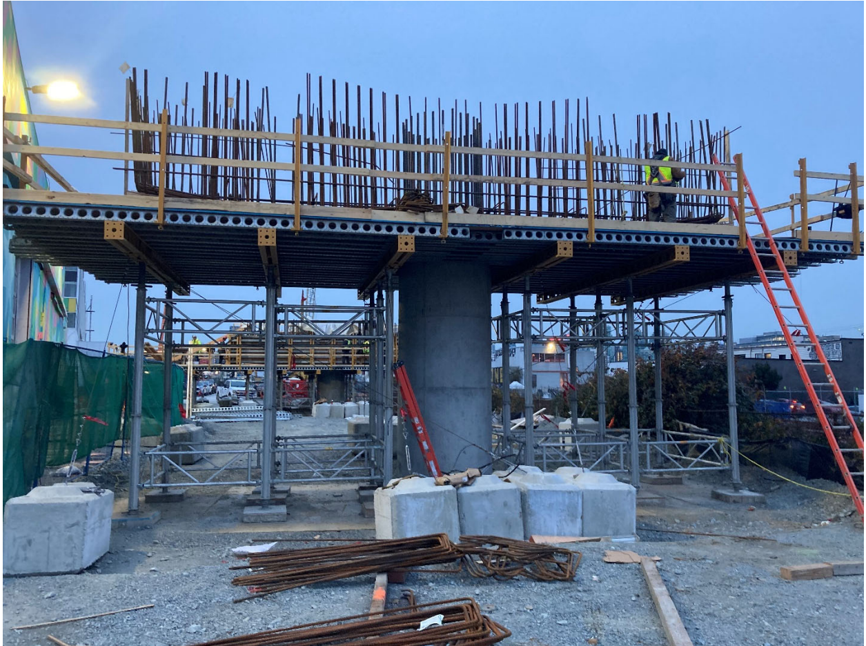
Figure 1: Elevated Guideway: Installation of pier caps on the caissons to support the elevated guideway.
