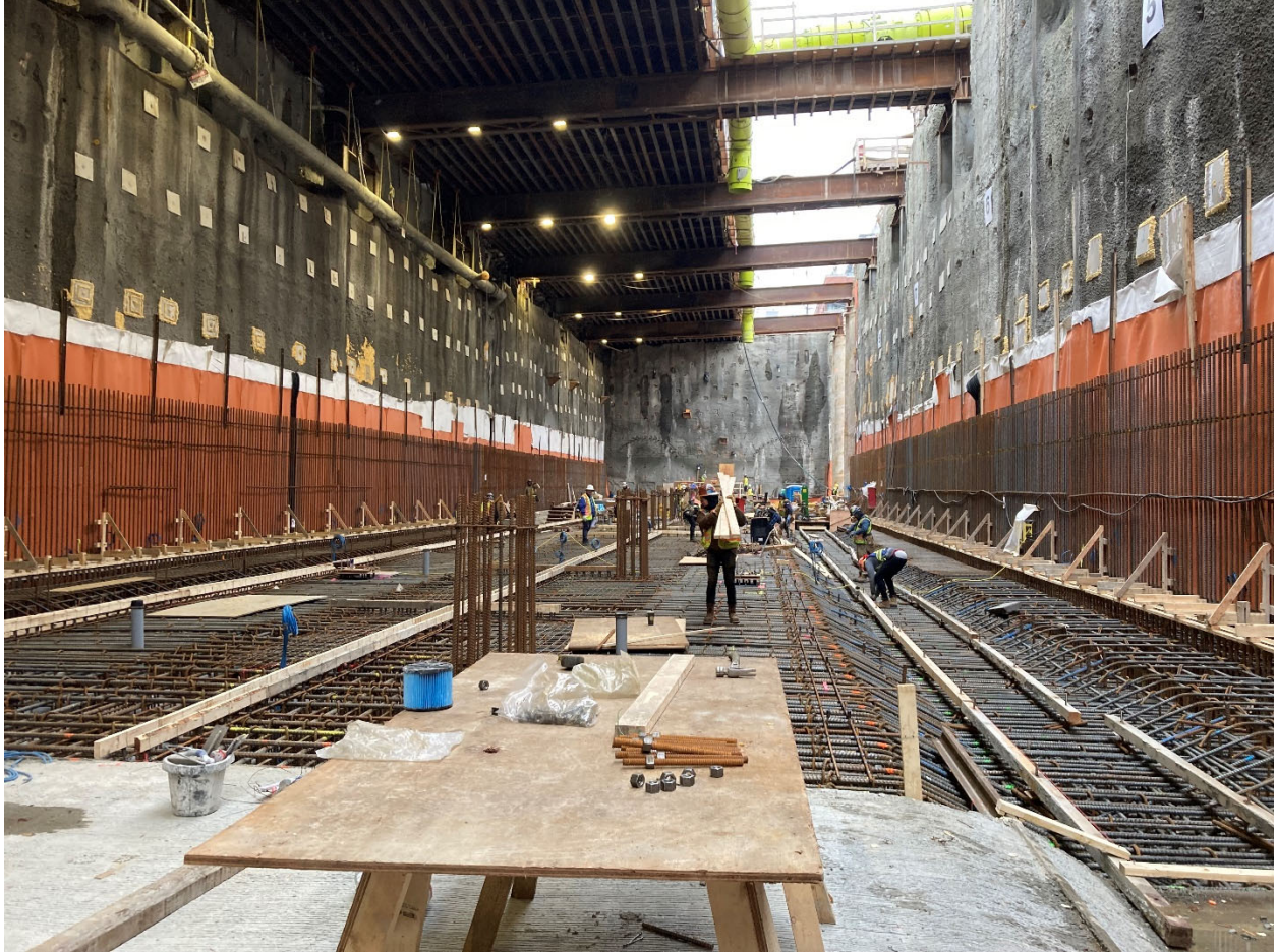
Figure 3: Mount Pleasant Station: Progressing with the installation of rebar and conduit for the station box base slab.
