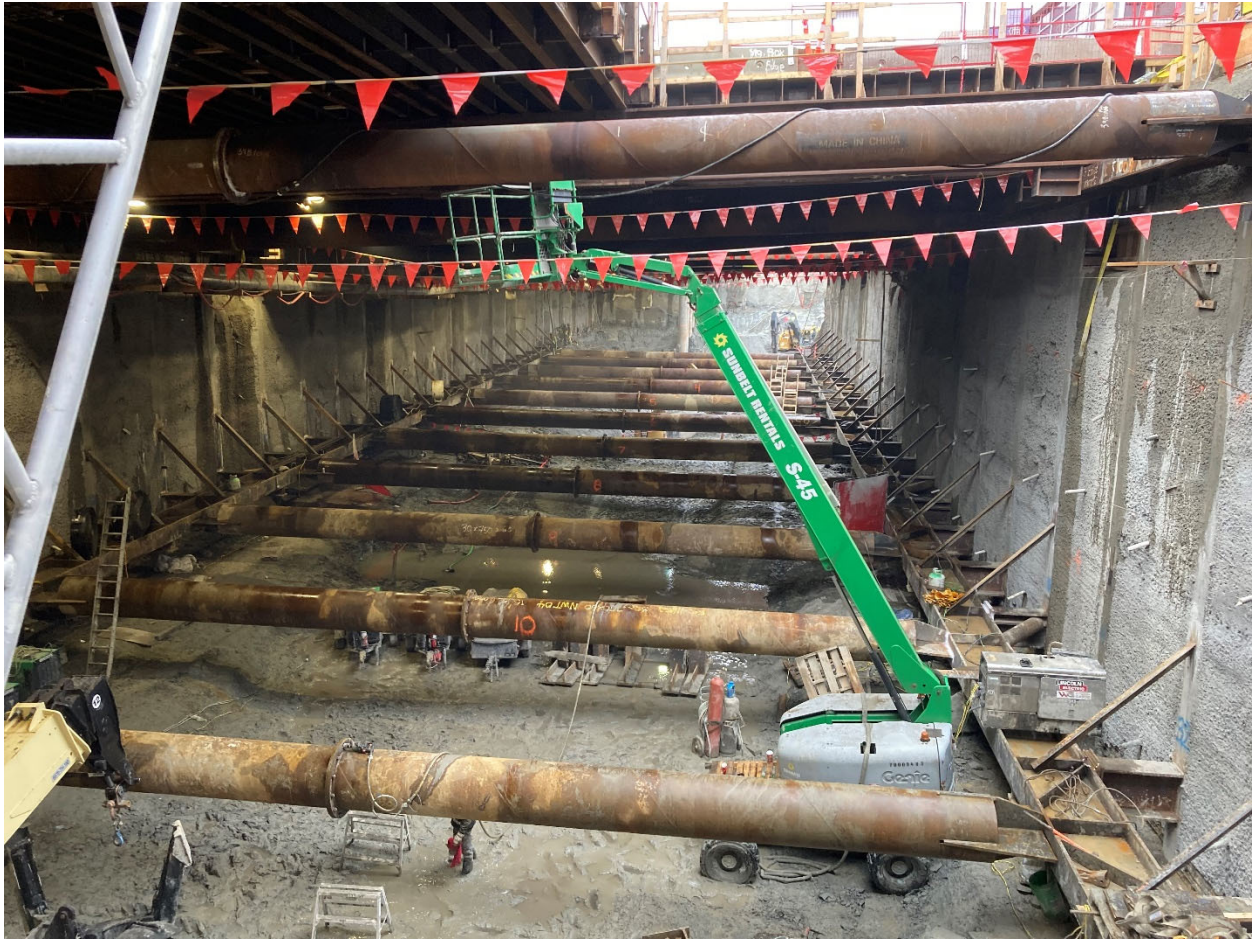
Figure 5: Oak-VGH Station: Progressing with the installation of structural supports for the station box.
