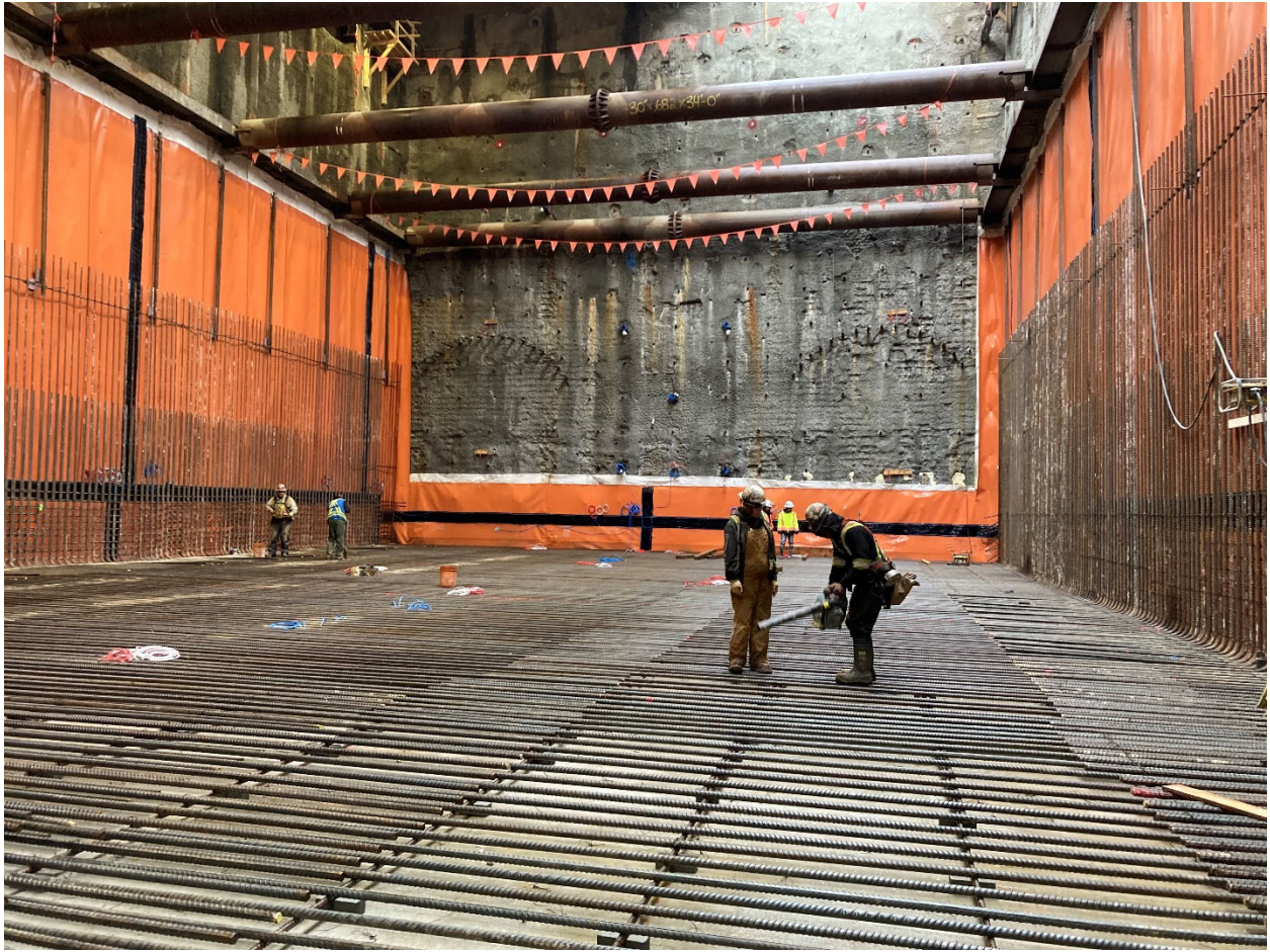
Figure 4: Broadway-City Hall Station: Progressing with the installation of waterproofing and rebar within the crossover section.
