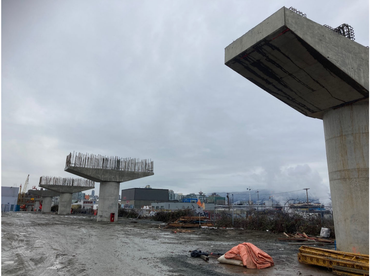
Figure 1: Elevated Guideway: Installation of pier caps on the columns to support the elevated guideway.
