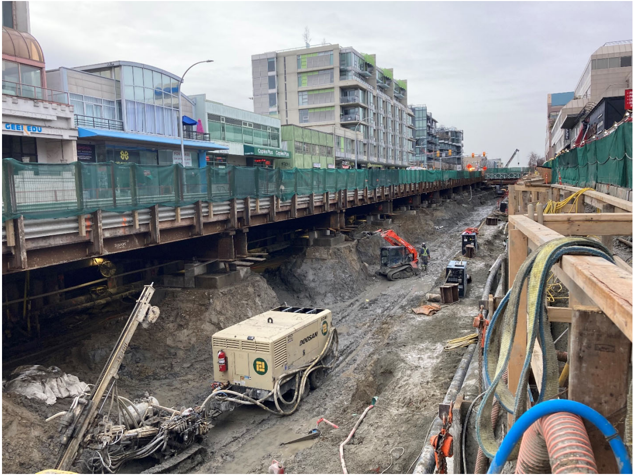
Figure 7: Arbutus Station: Progressing with shallow excavation to complete the traffic deck.
