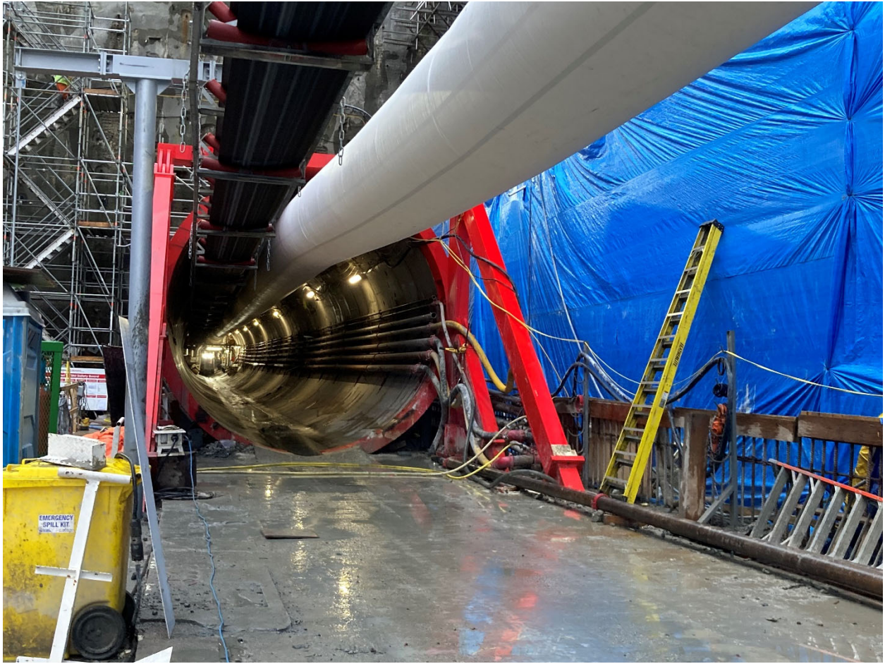
Figure 2: Great Northern Way-Emily Carr Station: TBM “Phyllis” progressing with the boring of the inbound tunnel to Mount Pleasant.
