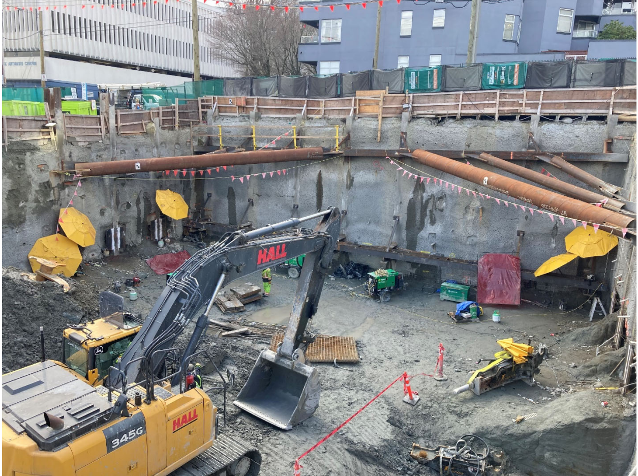
Figure 5: Oak-VGH Station: Progressing with the installation of a shoring support structure for the headhouse excavation.
