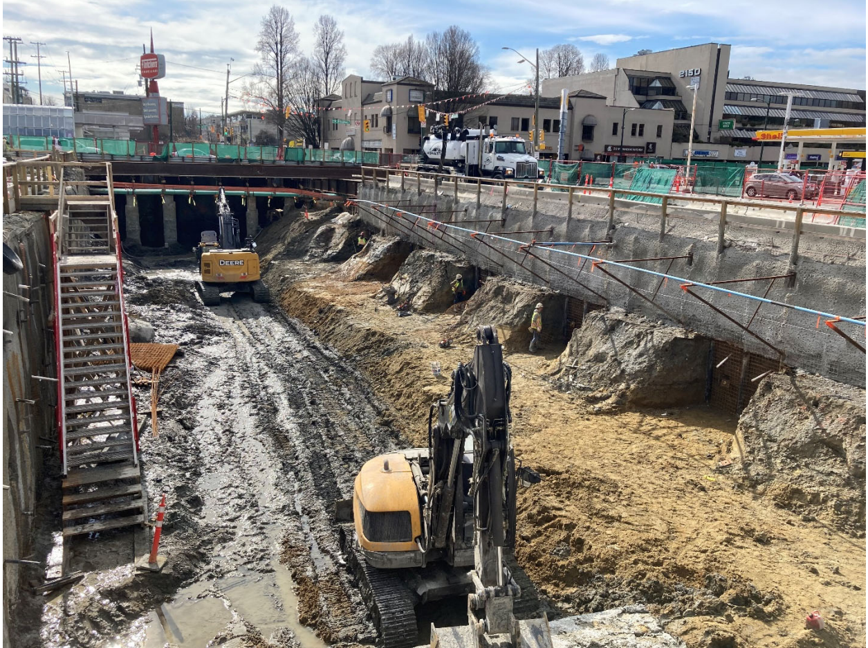
Figure 7: Arbutus Station: Progressing with the excavation and shoring for the headhouse.
