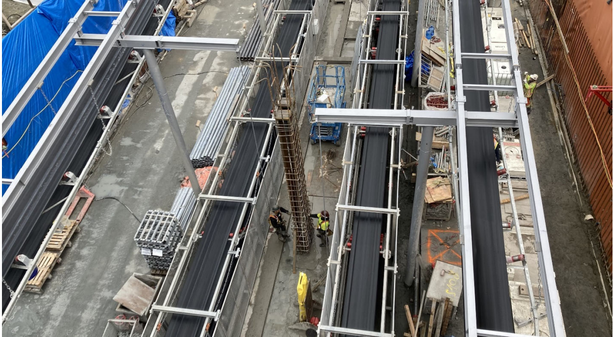
Figure 2: Great Northern Way-Emily Carr Station: Progressing with interior columns installation while the tunnel boring conveyor systems transports excavated material out of the tunnels.
