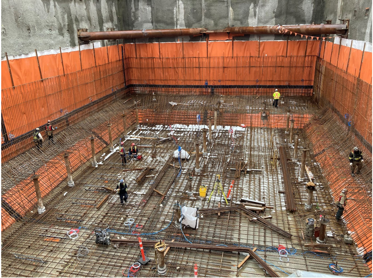
Figure 3: Mount Pleasant Station: Progressing with the installation of rebar and conduit for the headhouse base slab.
