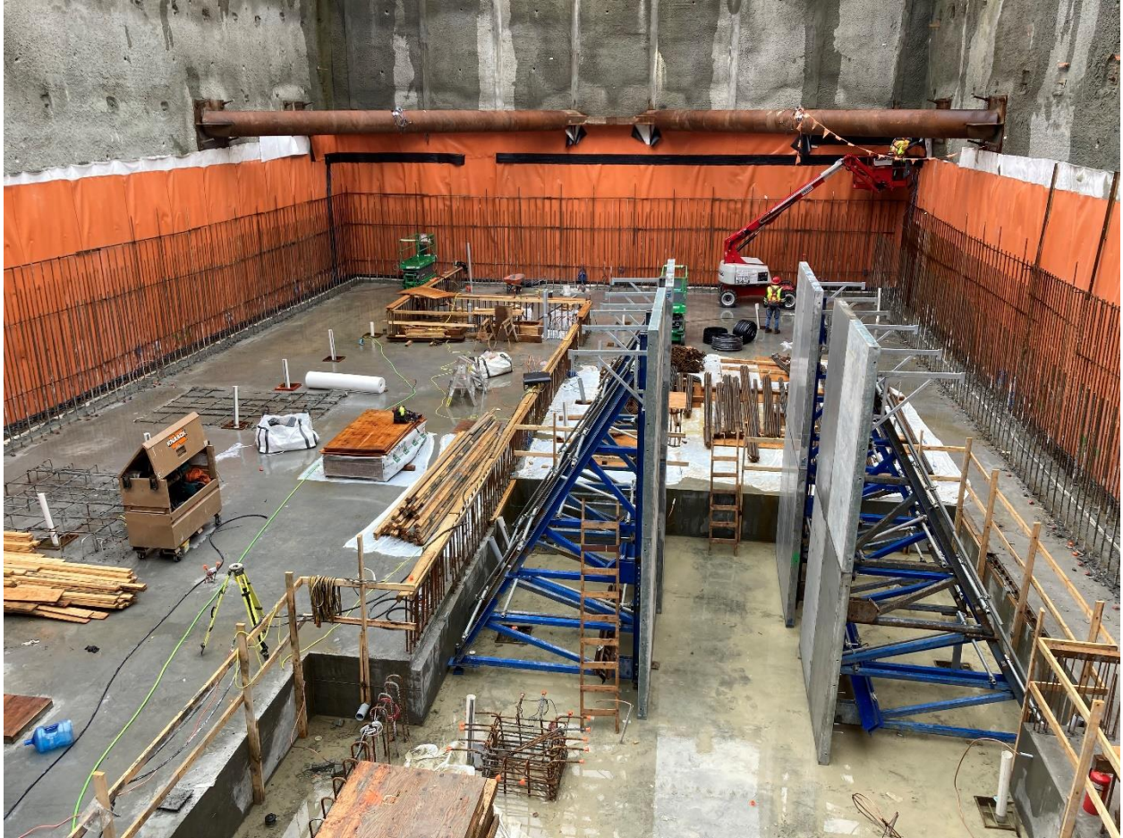
Figure 3: Mount Pleasant Station: With the base slab poured, the installation of waterproofing, rebar, and wall forms was in progress within the headhouse.
