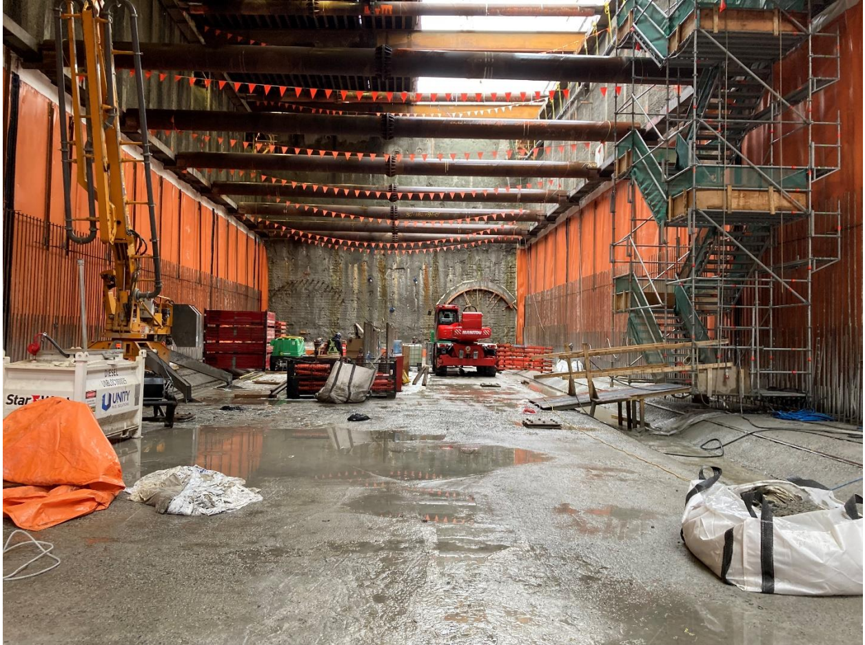
Figure 4: Broadway-City Hall Station: Within the Crossover, preparation to receive Outbound TBM Elsie was in progress.
