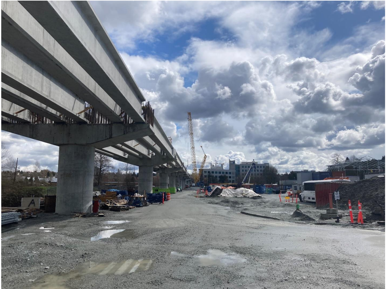
Figure 1: Elevated Guideway: Progressing with the installation of girders for the elevated guideway structure.
