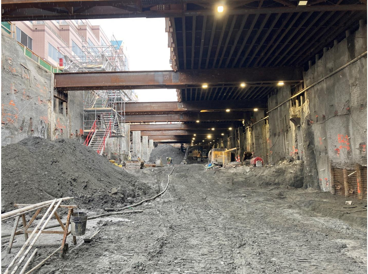
Figure 7: Arbutus Station: Progressing with the excavation and shoring for the station box.
