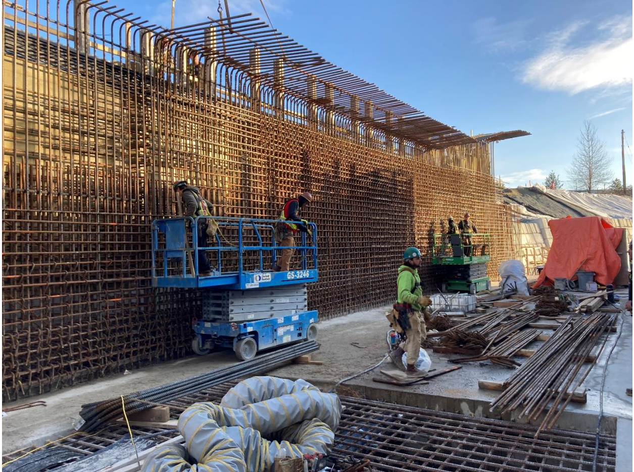
Figure 2: Great Northern Way-Emily Carr Station: Progressing with the installation of rebar and wall forms for the transition box.
