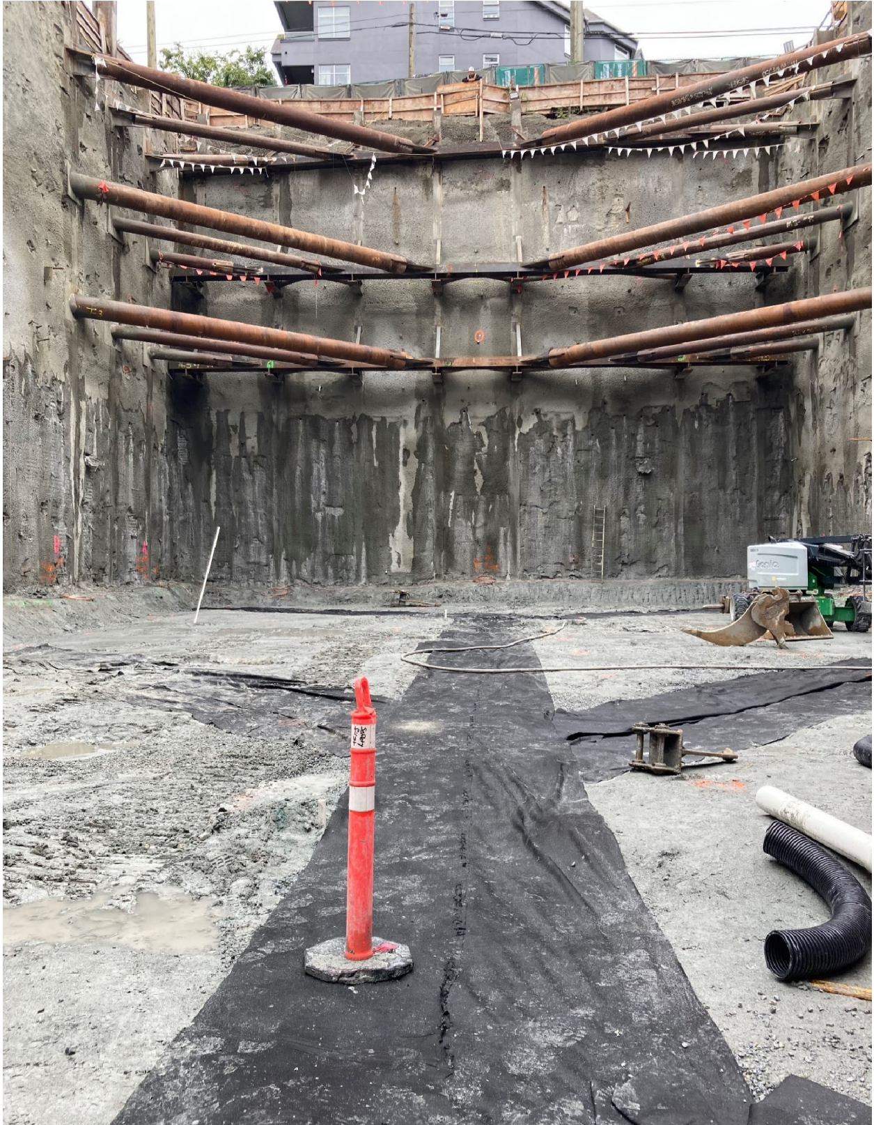
Figure 5: Oak-VGH Station: Headhouse excavation has been completed.
