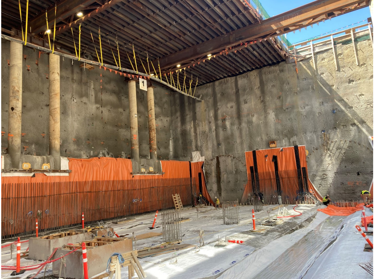
Figure 6: South Granville Station: Base slab poured at the west end of the station box.
