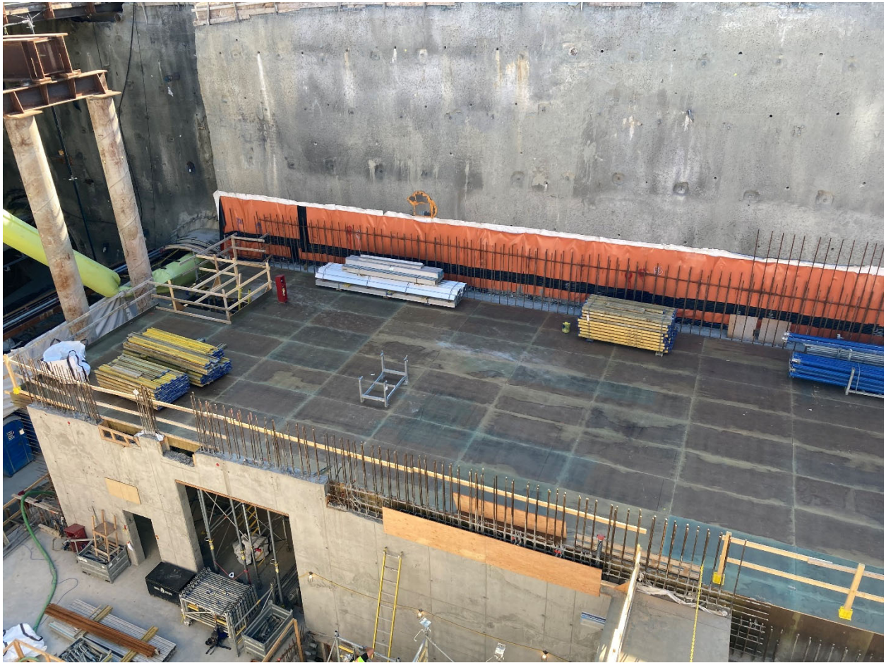
Figure 3: Mount Pleasant Station: Progressing with the installation of scaffolding and decking for the concourse slab in the headhouse.
