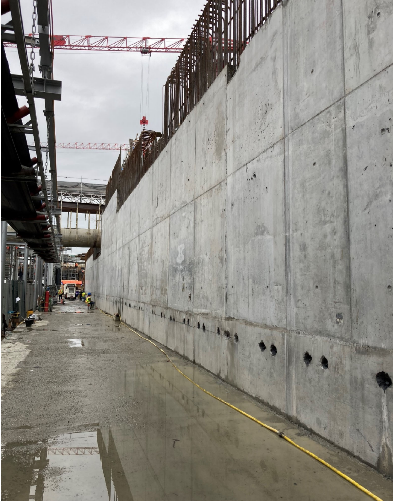
Figure 2: Great Northern Way-Emily Carr Station: Progressing with the construction of walls for the station box.
