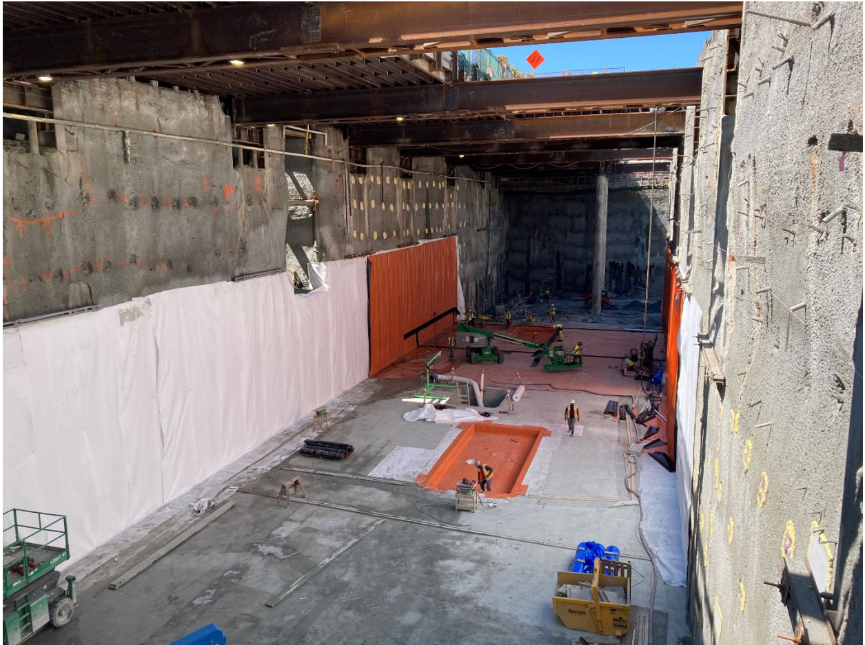
Figure 7: Arbutus Station: Progressing with the installation of waterproofing in the station box.
