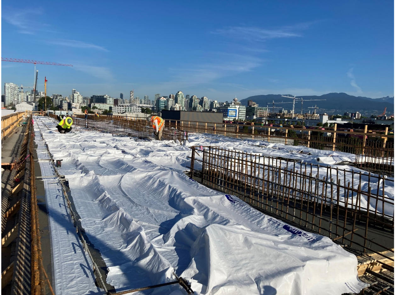
Figure 1: Elevated Guideway: Installation of the cast-in-place concrete bottom slab on the elevated guideway structure.
