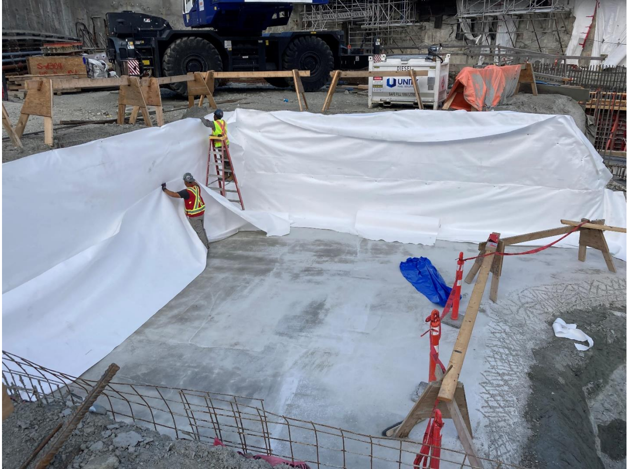
Figure 2: Great Northern Way-Emily Carr Station: Progressing with the installation of waterproofing within the headhouse excavation.
