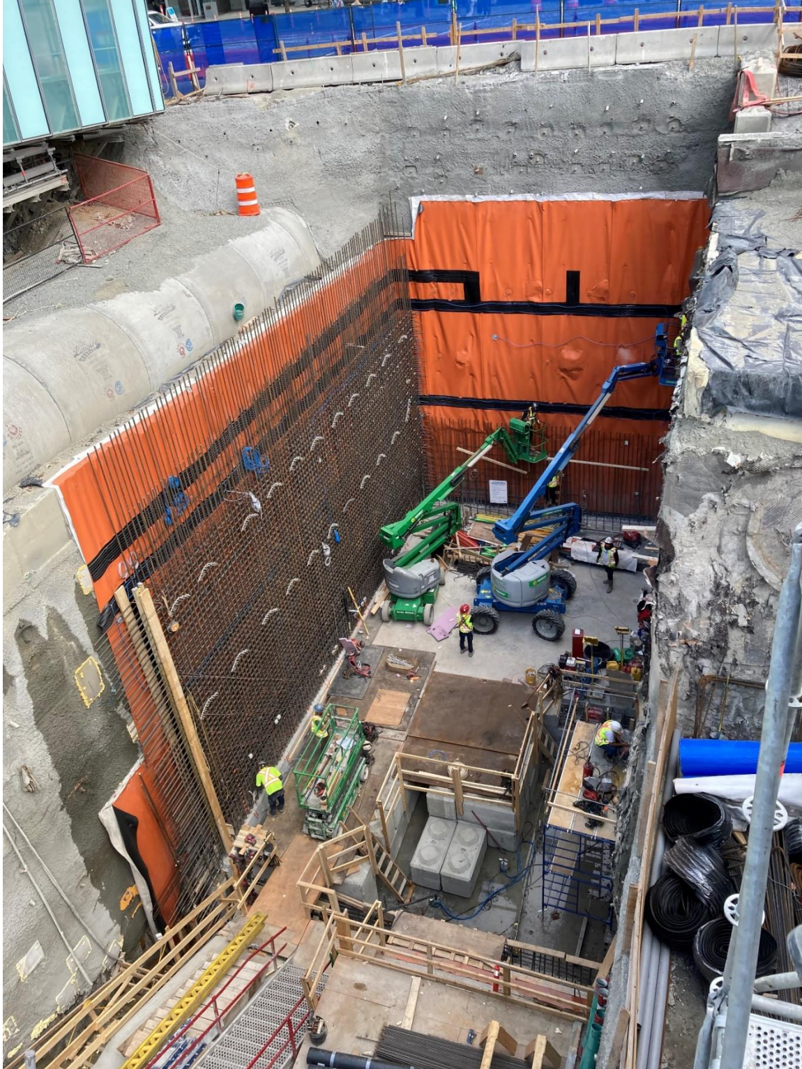
Figure 4: Broadway-City Hall Station: Progressing with rebar installation to build the walls of the passenger connections between the Canada Line and future Millennium Line platforms.
