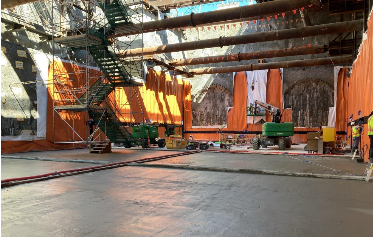
Figure 6: South Granville Station: Progressing with the base slab installation. Base slab poured at the west end of the station box.
