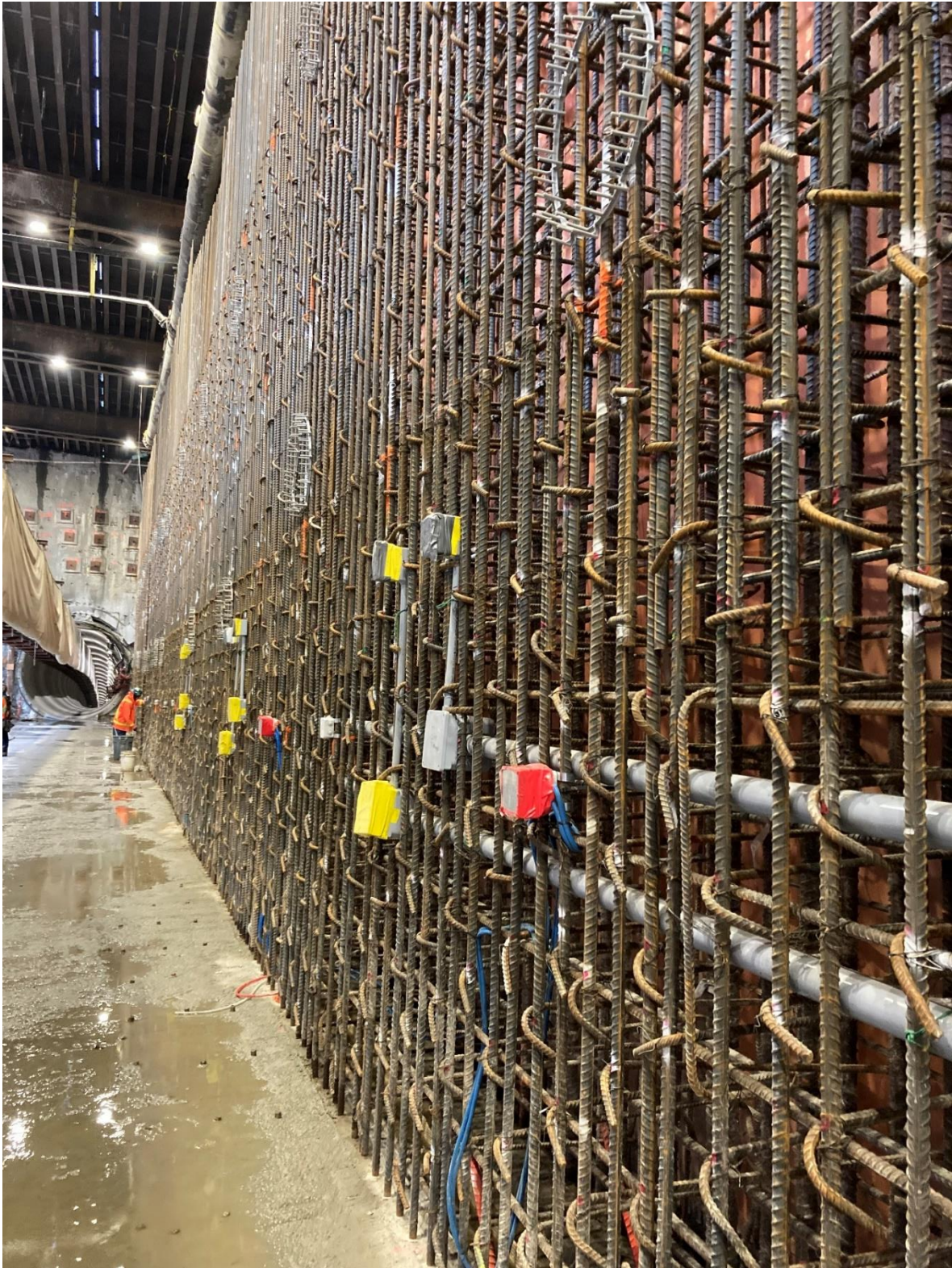
Figure 3: Mount Pleasant Station: Progressing with the installation of rebar and electrical conduits for the station walls.
