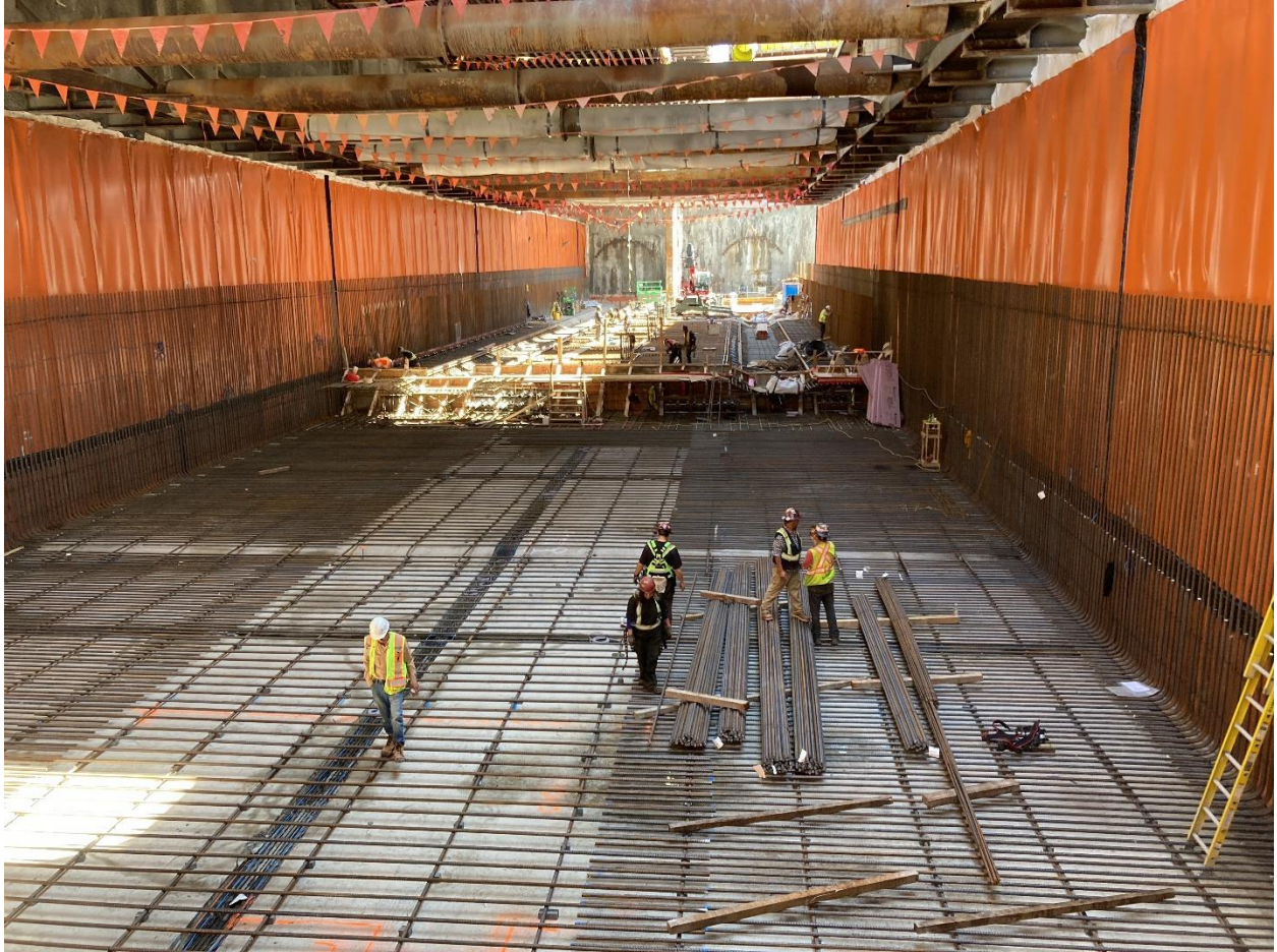
Figure 5: Oak-VGH Station: Preparations for next base slab concrete pour.
