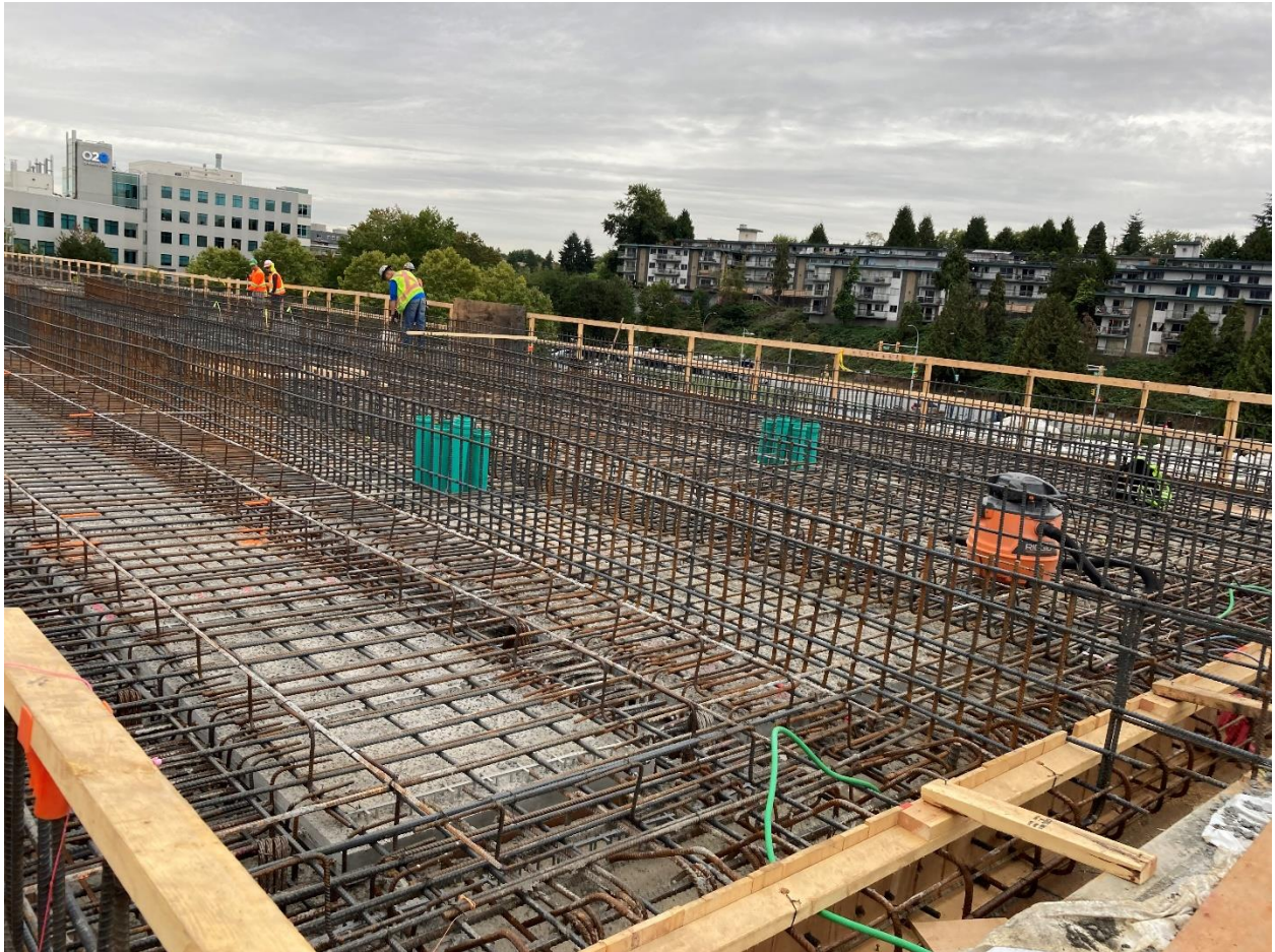
Figure 1: Elevated Guideway: Progressing with the installation of rebar for the elevated guideway deck.
