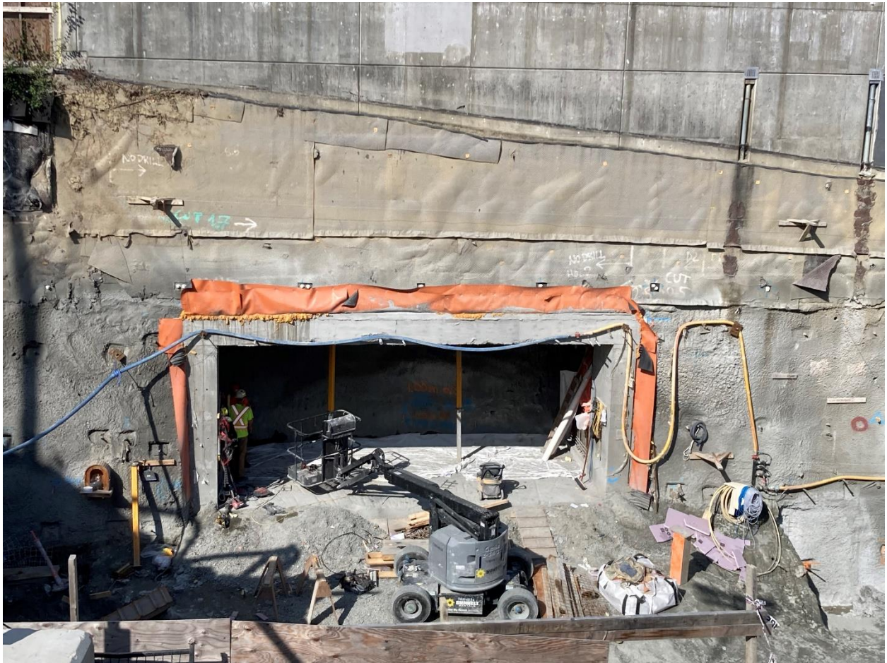
Figure 4: Broadway-City Hall Station: Progressing with waterproofing and rebar installation for the south underpass.
