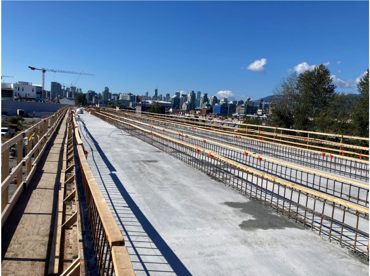
Figure 1: Elevated Guideway: Progressing with the installation of a base layer slab for the elevated guideway deck.
