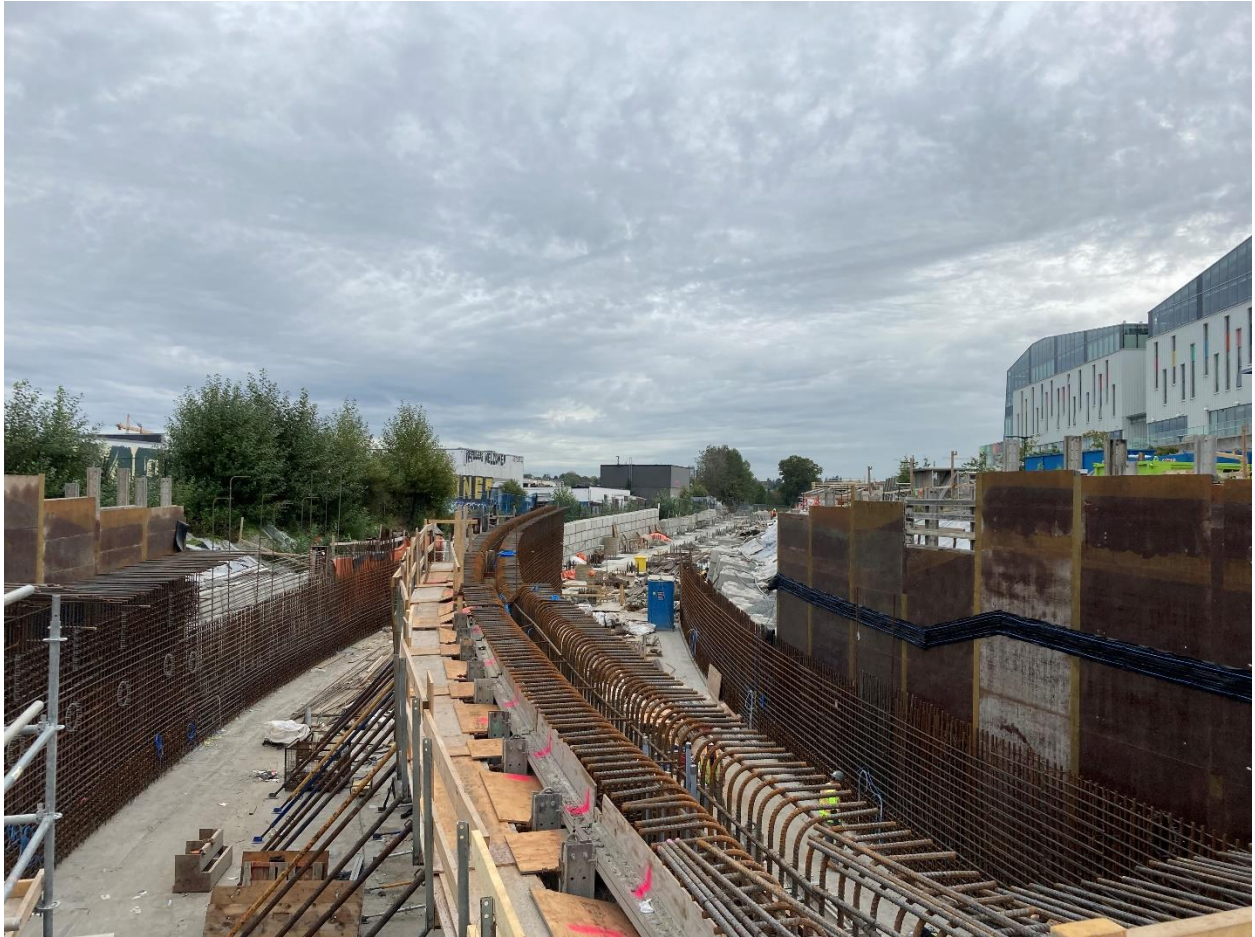
Figure 2: Great Northern Way-Emily Carr Station: Progressing with the installation of center and perimeter transition box walls.
