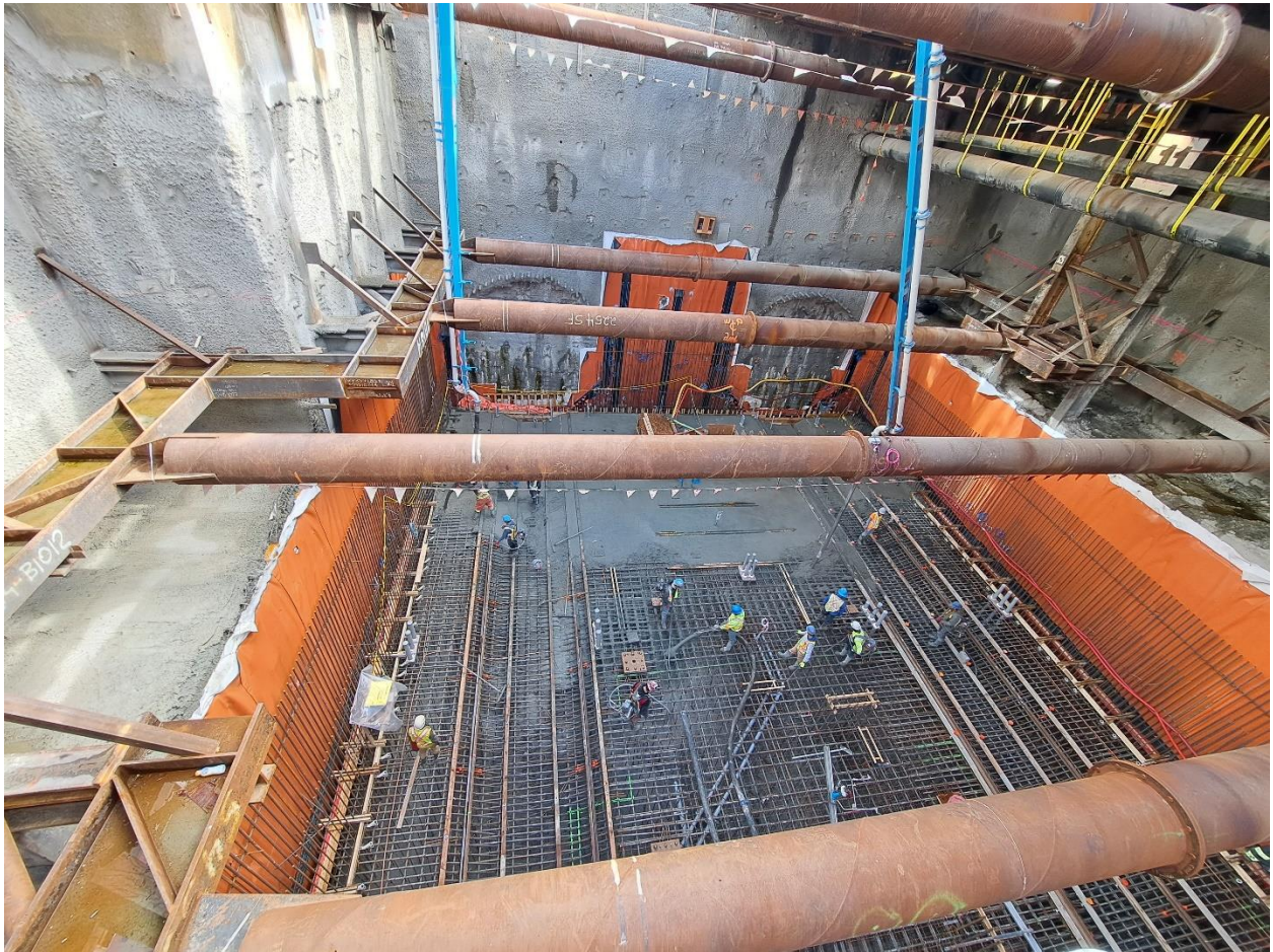
Figure 6: South Granville Station: Progressing with the base slab installation at the east end of the station box.
