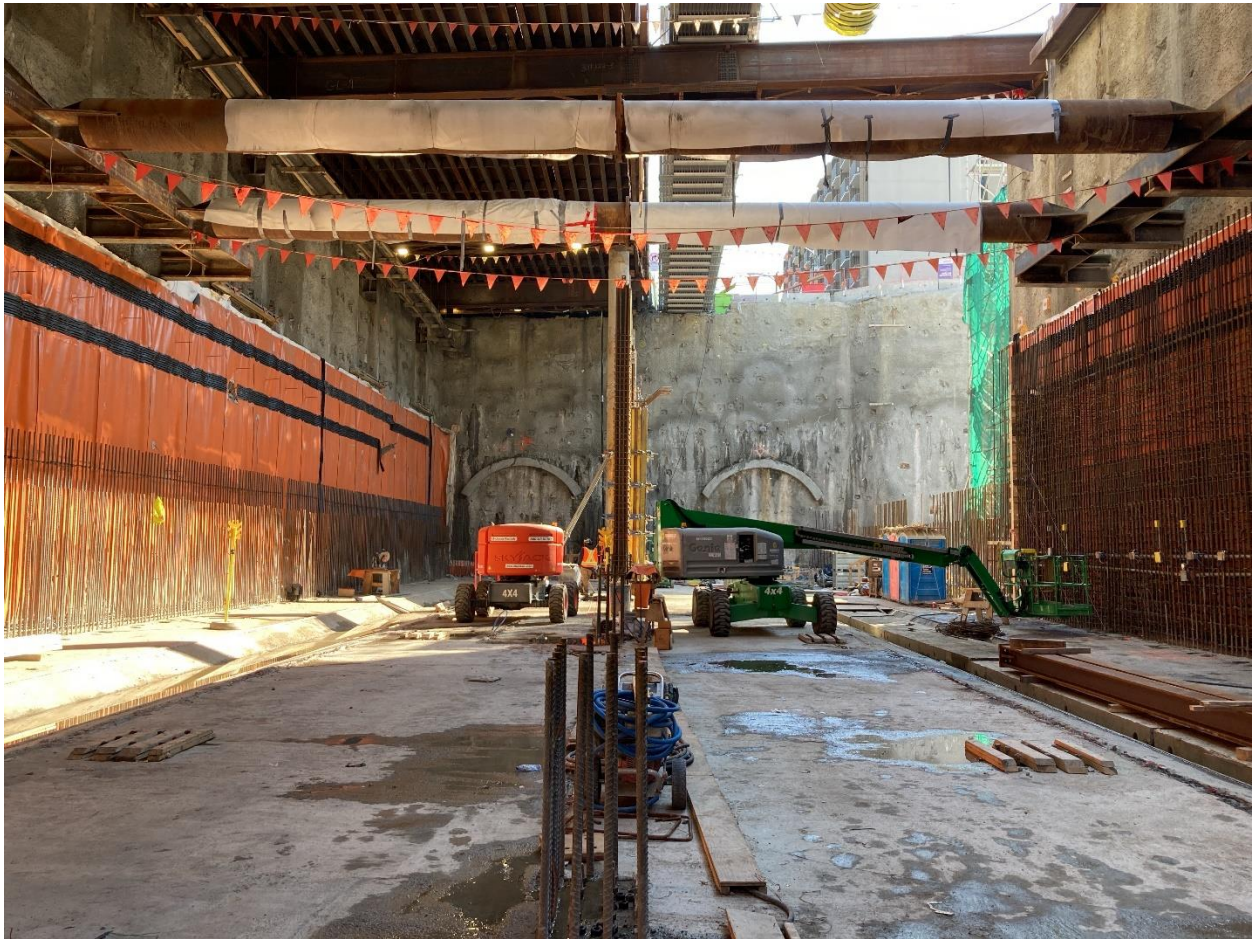
Figure 5: Oak-VGH Station: Preparation for the breakthrough of Inbound TBM Phyllis.
