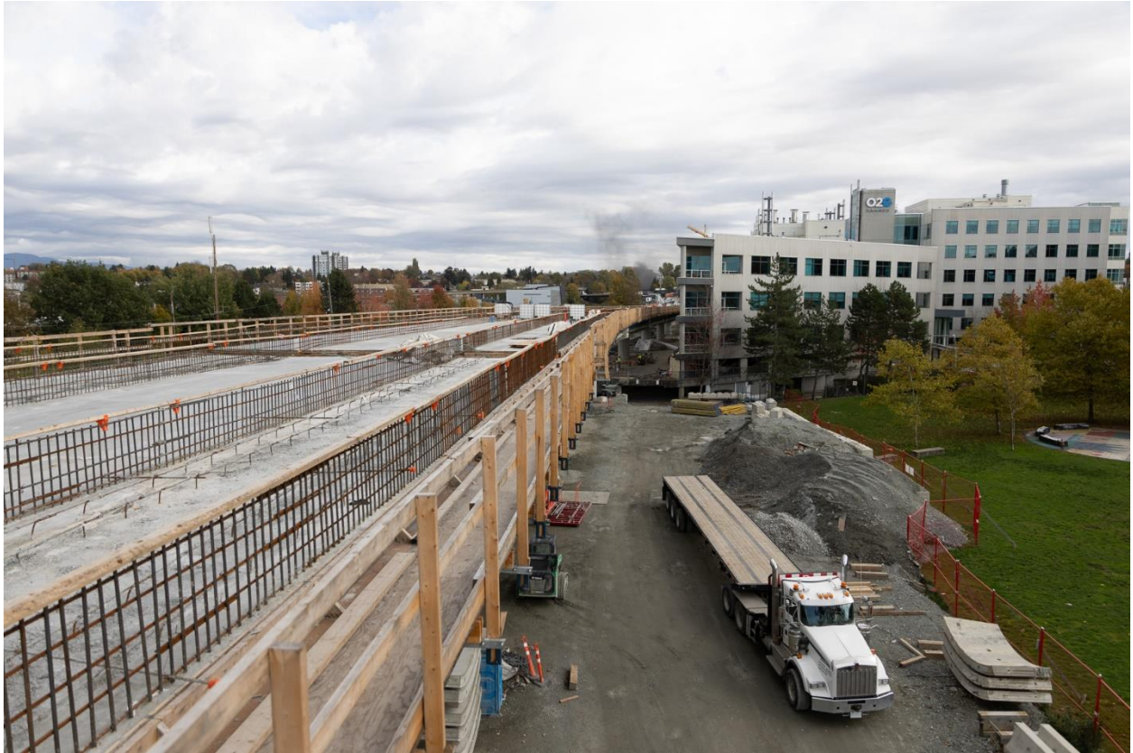
Figure 1: Elevated Guideway: Progressing with the installation of concrete for the elevated guideway deck.
