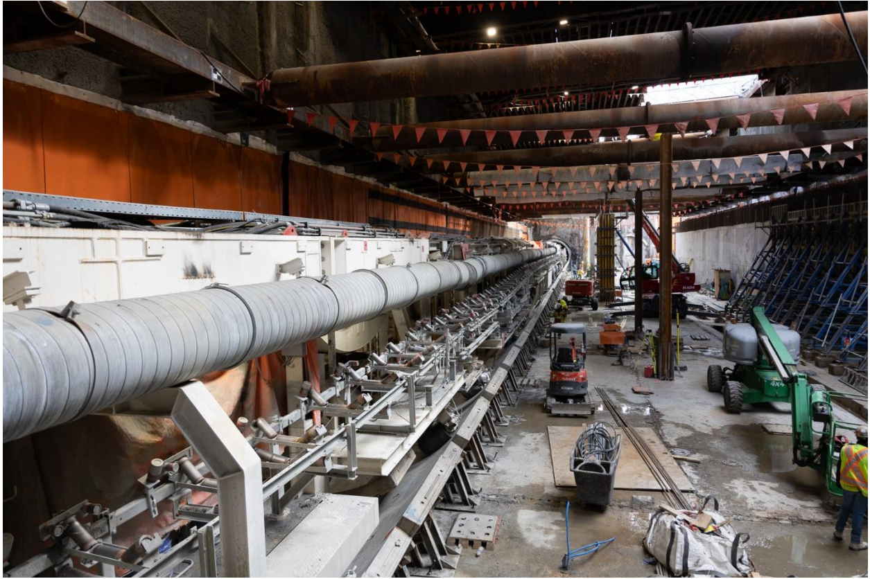
Figure 5: Oak-VGH Station: Preparation for the relaunch of Inbound TBM Phyllis.
