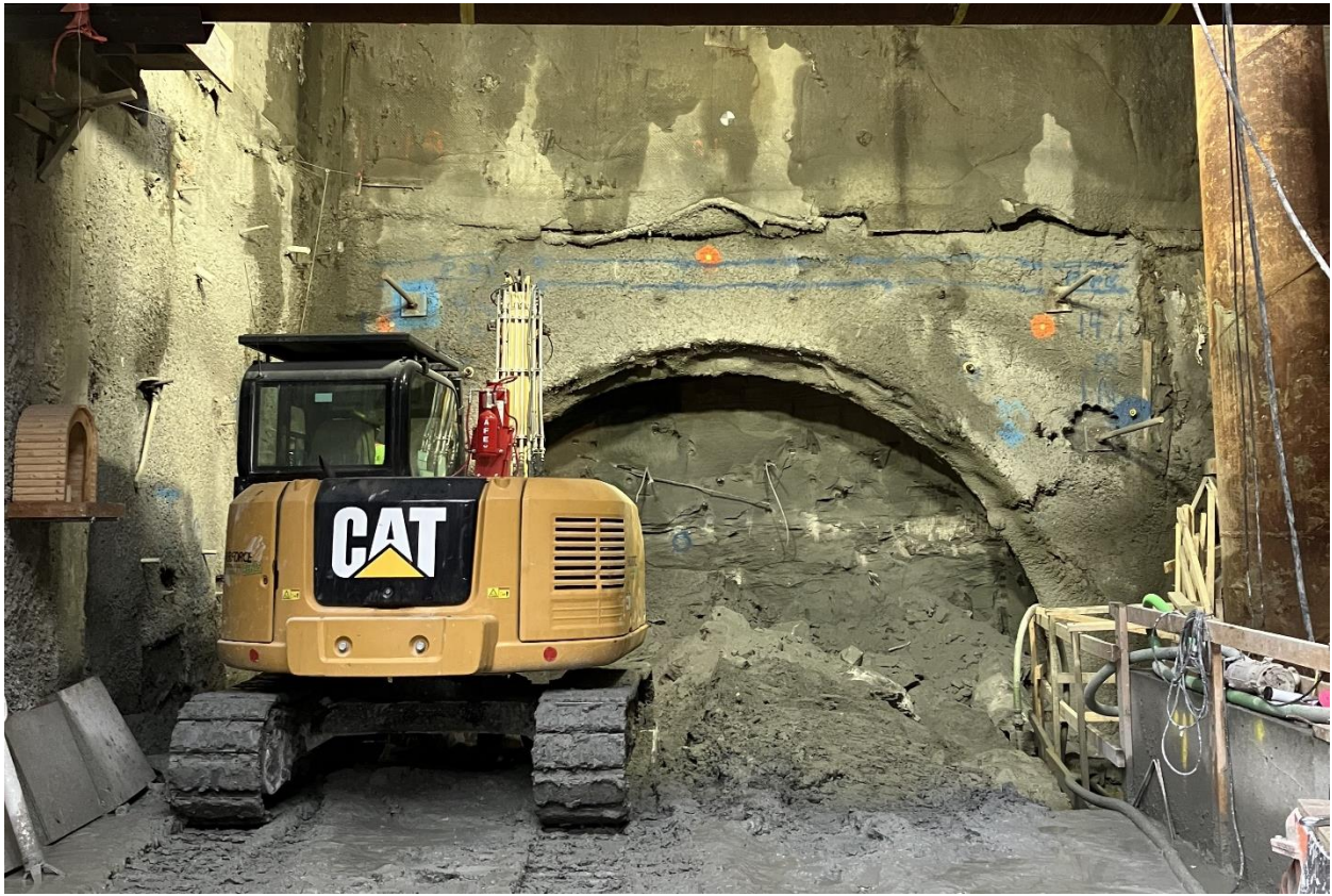
Figure 4: Broadway-City Hall Station: Progressing with excavating the mined tunnel for the passenger connection to the southbound platform of the Canada Line.
