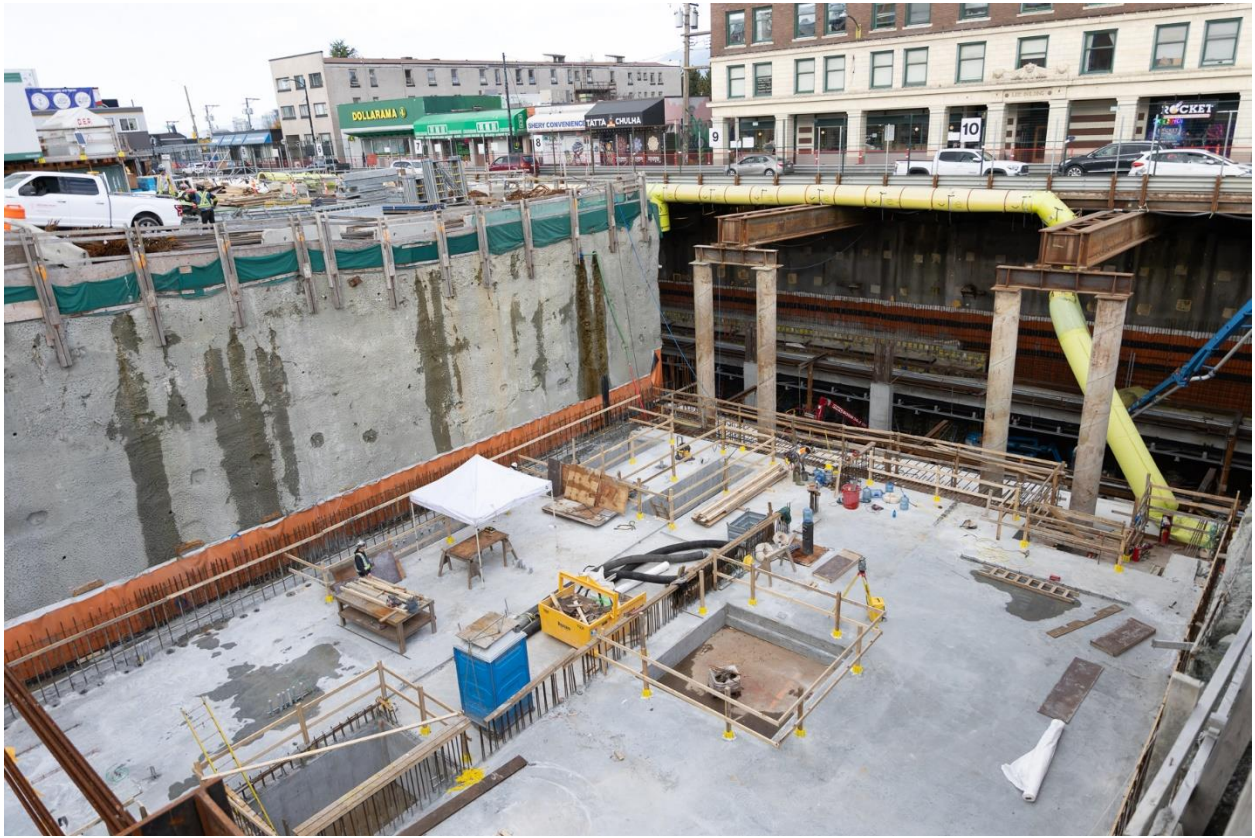
Figure 3: Mount Pleasant Station: Progressing with the installation of the concourse slab in the headhouse and station area.
