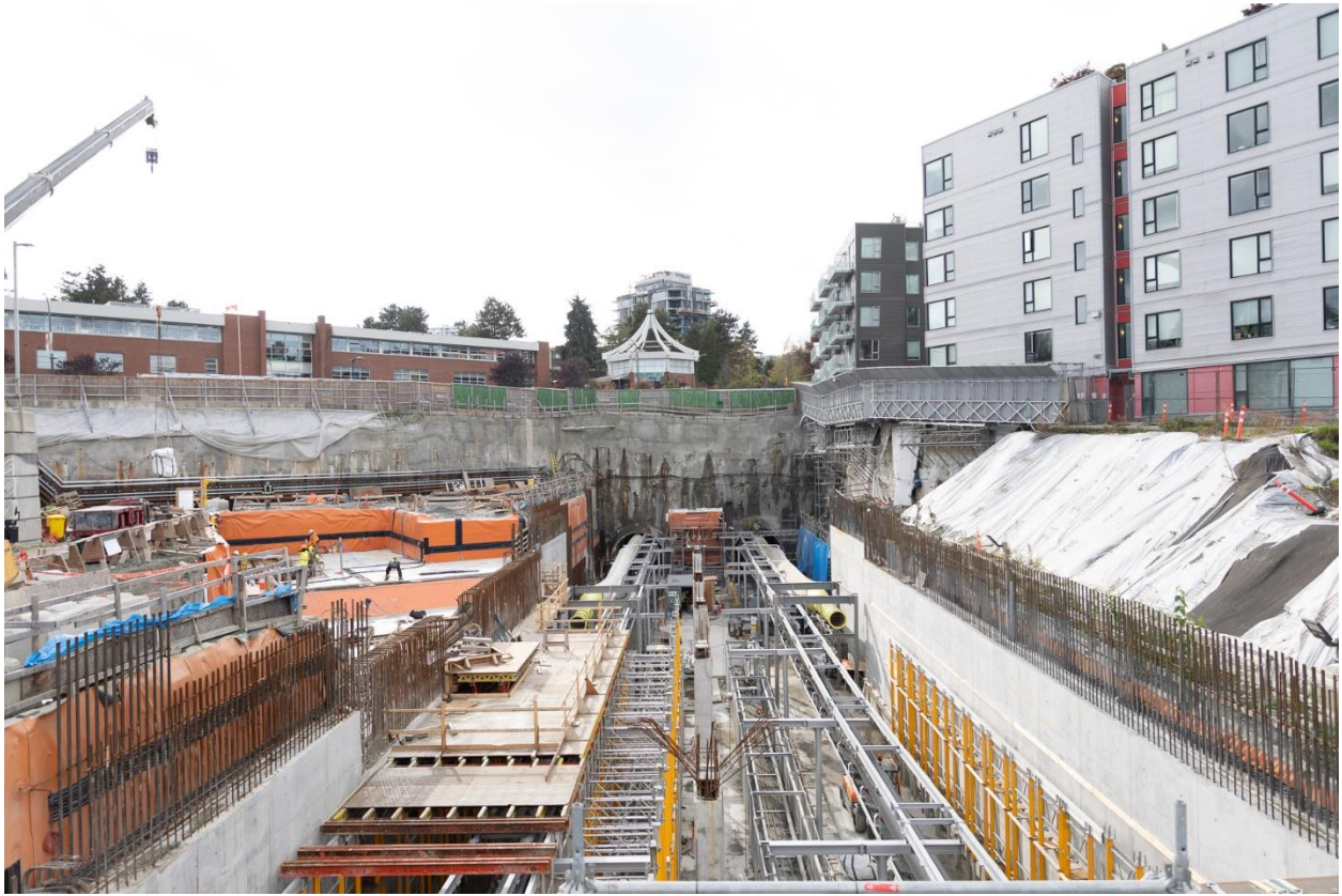
Figure 2: Great Northern Way-Emily Carr Station: Progressing with installation of scaffolding to construct the concourse slab in the station area.
