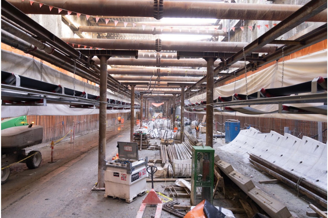
Figure 4: Broadway-City Hall Station: Progressing with the removal of temporary tunnel liner segments and infilling the TBM cradle slab.
