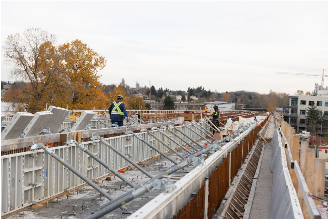
Figure 1: Elevated Guideway: Progressing with concrete pours to construct the parapets.
