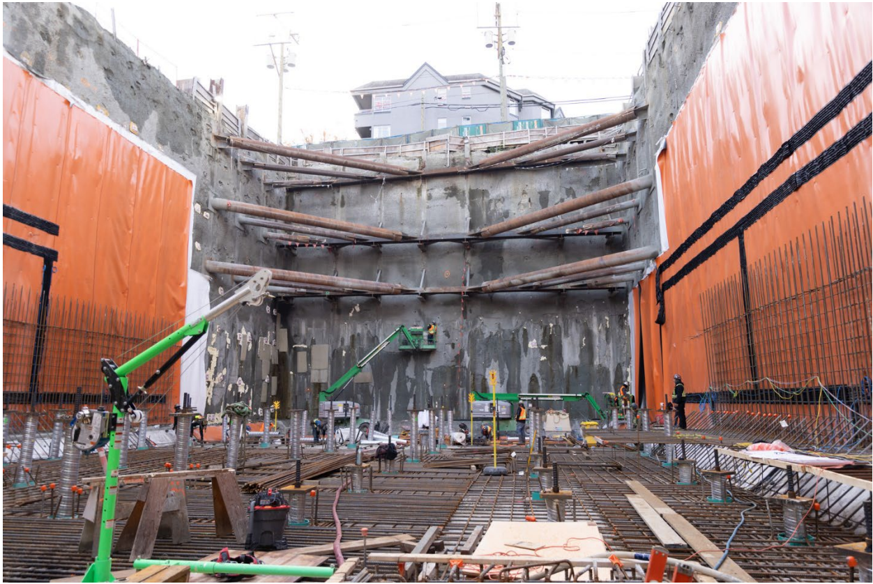
Figure 5: Oak-VGH Station: Progressing with the installation of rebar for the headhouse base slab.
