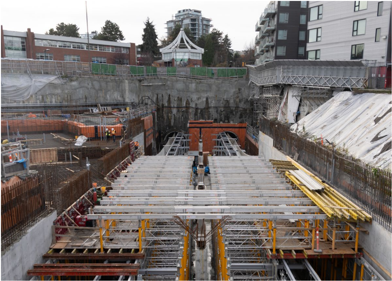
Figure 2: Great Northern Way-Emily Carr Station: Progressing with installation of rebar for the headhouse base slab.
