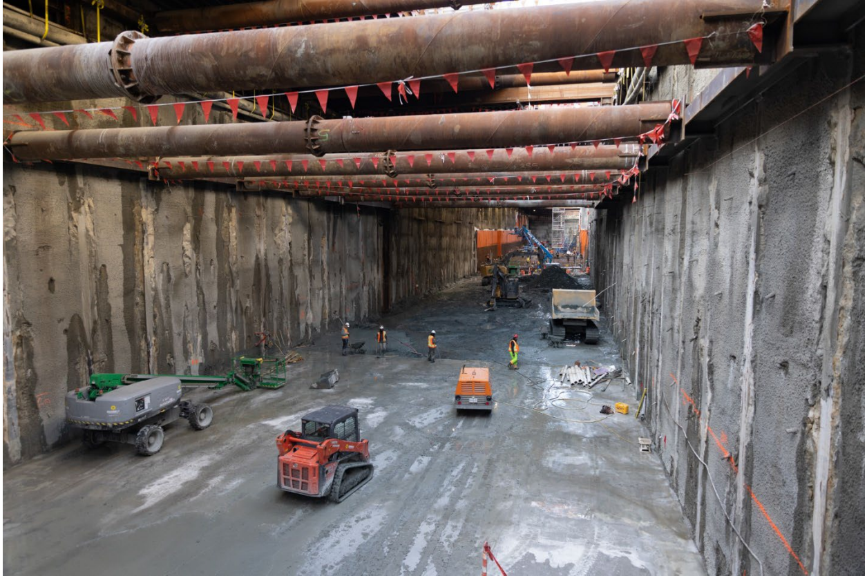
Figure 7: Arbutus Station: Excavation completed in the crossover area.
