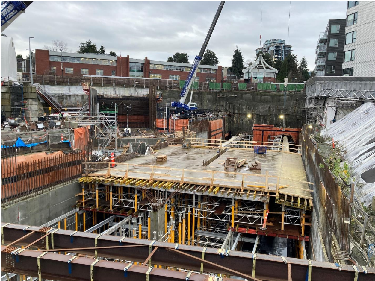
Figure 2: Great Northern Way-Emily Carr Station: Progressing with installation of rebar for the concourse level walls in the headhouse and preparing the concourse level floor in the station box.
