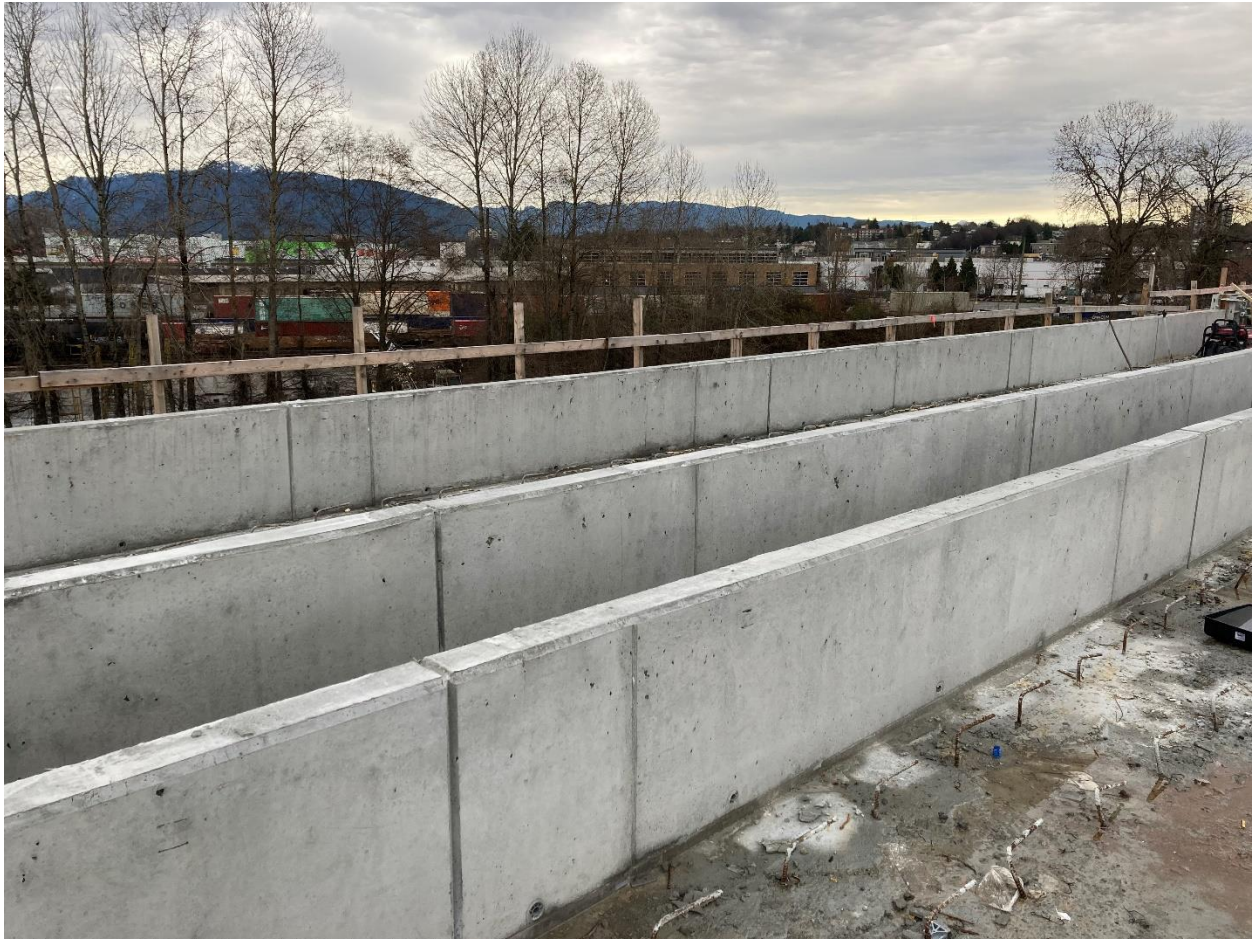
Figure 1: Elevated Guideway: Progressing with concrete pours to construct the parapets.
