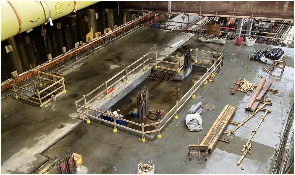
Figure 3: Mount Pleasant Station: Progressing with the installation of the concourse slab in the station area.
