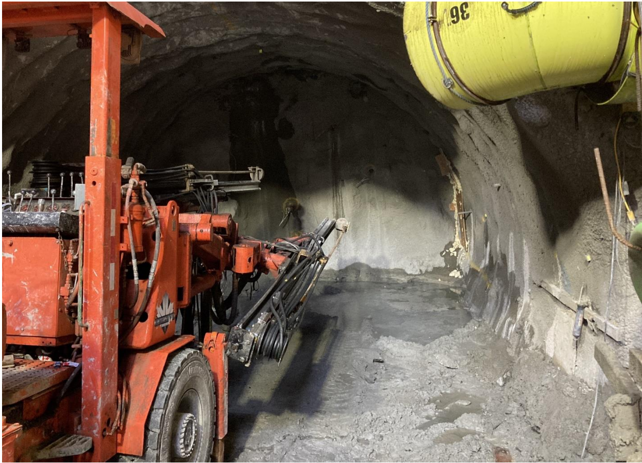
Figure 4: Broadway-City Hall Station: Progressing with excavation of the mined tunnel for the passenger connection to the southbound Canada Line platform.
