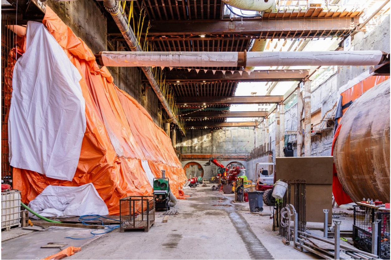
Figure 6: South Granville Station: Progressing with concrete pours for the station's south wall and preparations for relaunching TBM Phyllis.
