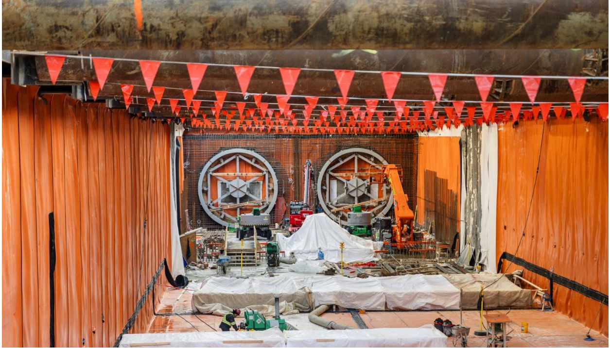
Figure 7: Arbutus Station: Progressing with preparations for the arrival of the tunnel boring machines.
