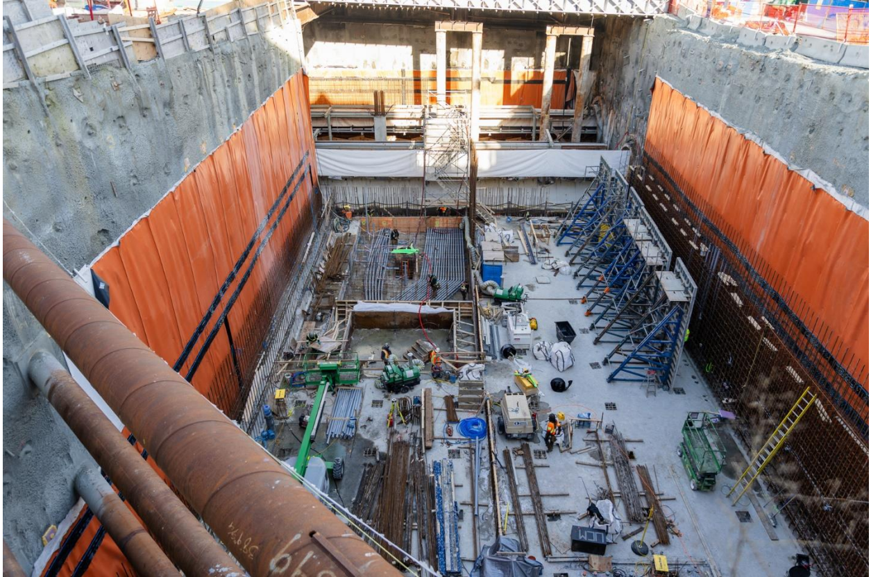
Figure 5: Oak-VGH Station: Progressing with rebar installation for the headhouse walls.
