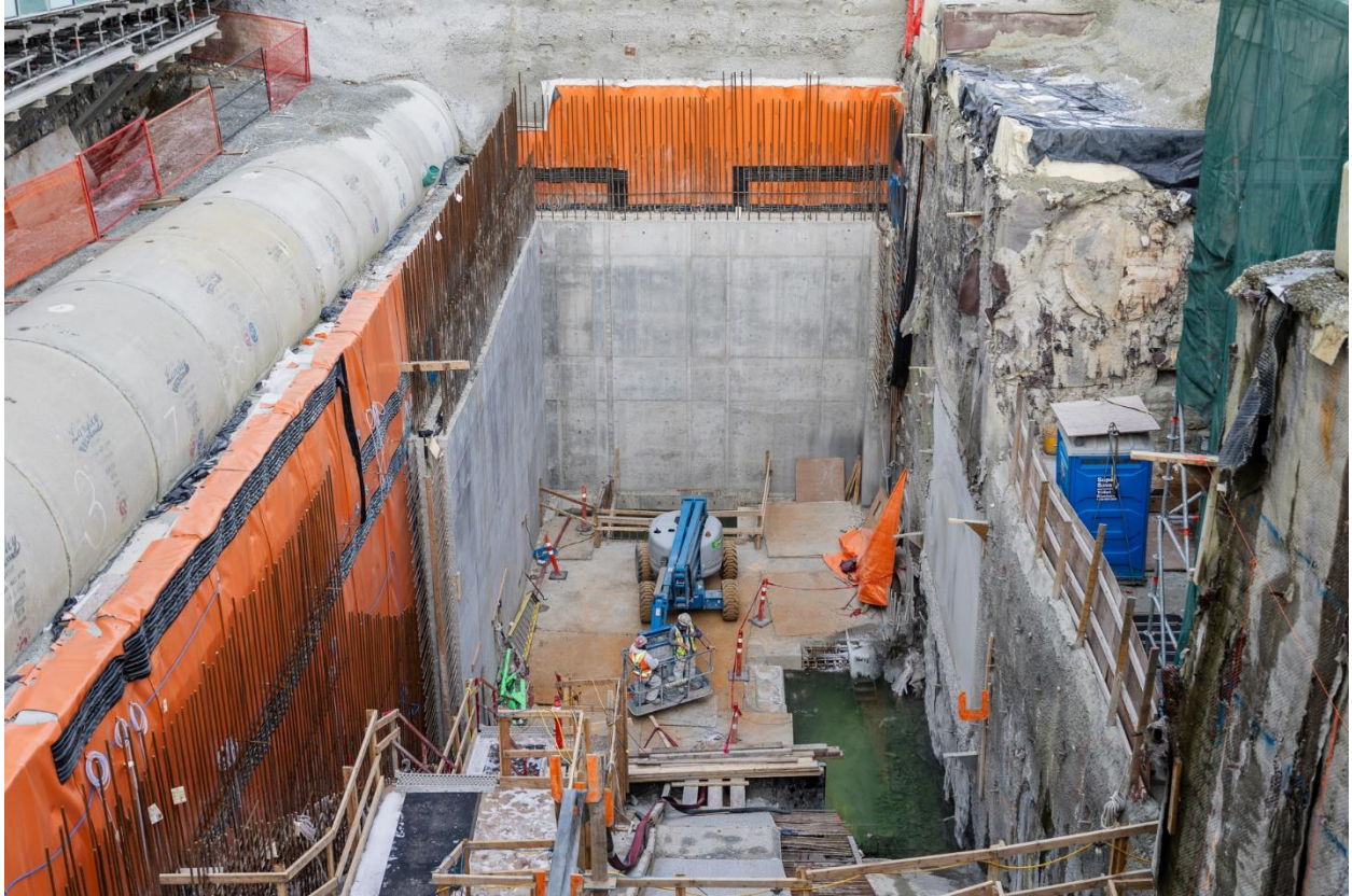
Figure 4: Broadway-City Hall Station: Progressing with preparations for construction of the eastern wall of the circulation shaft.
