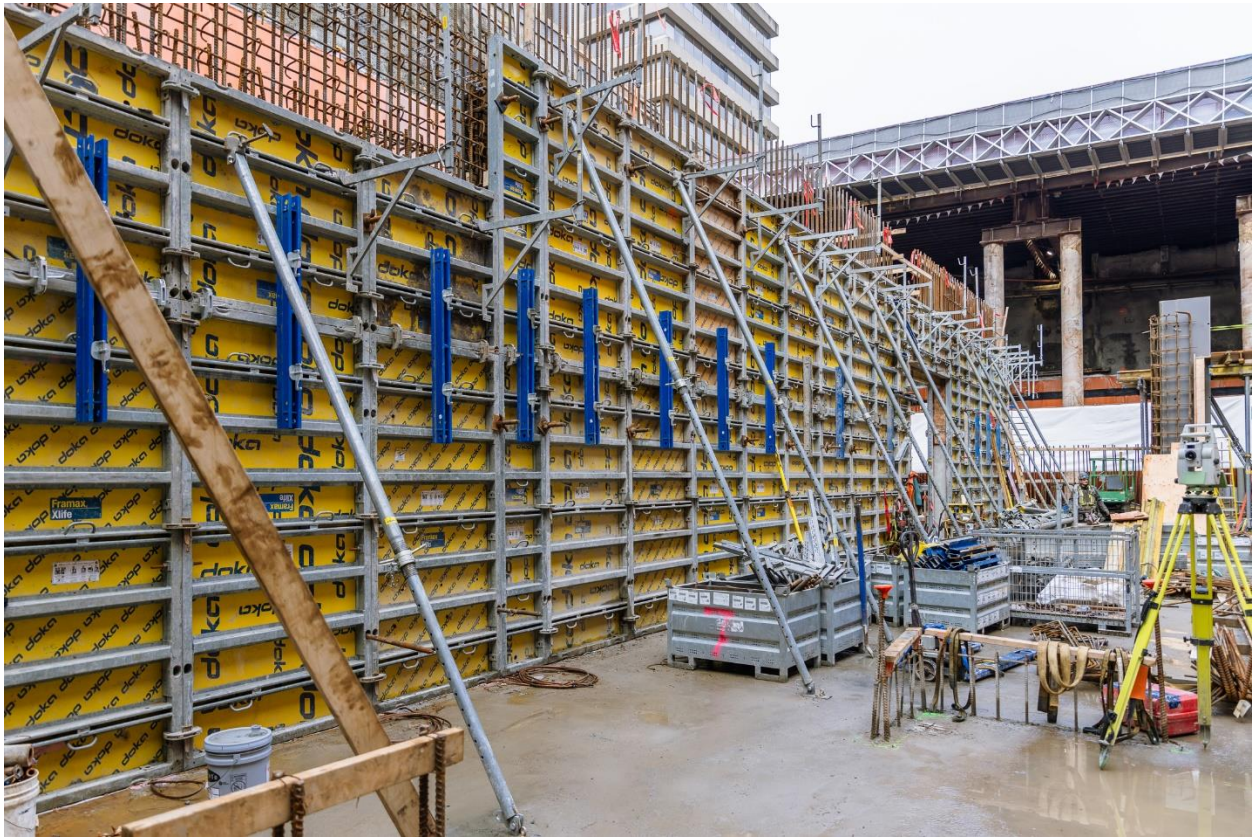
Figure 5: Oak-VGH Station: Progressing with concrete pours for the interior headhouse walls.
