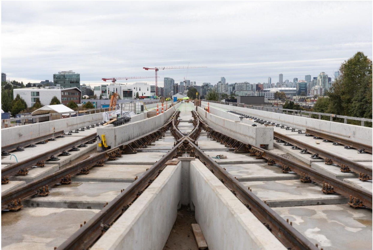
Figure 1: Elevated Guideway: Progressing with pouring the east track switch slab in the pocket track.
