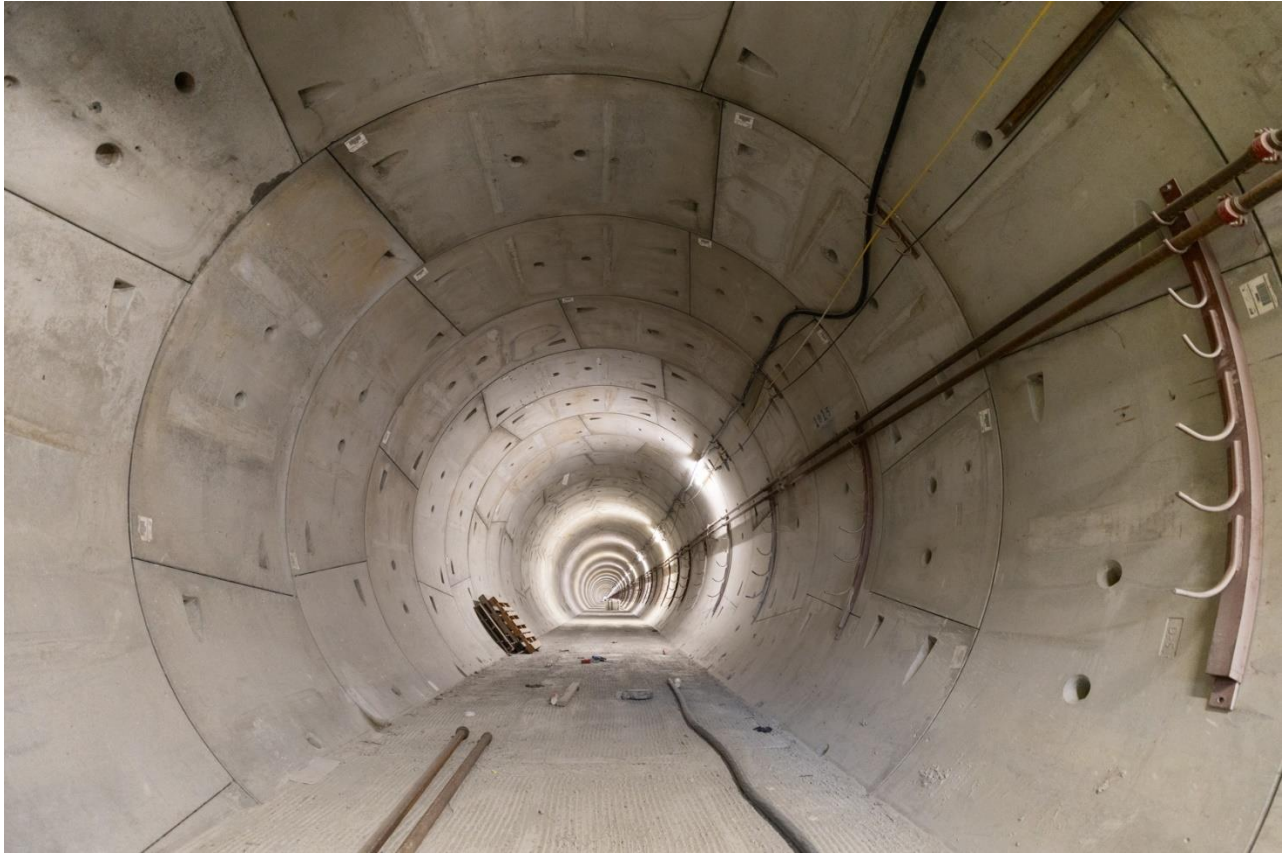
Figure 8: Tunnels: Completion of the invert slabs in the tunnels (outbound tunnel east of South Granville Station shown above).
