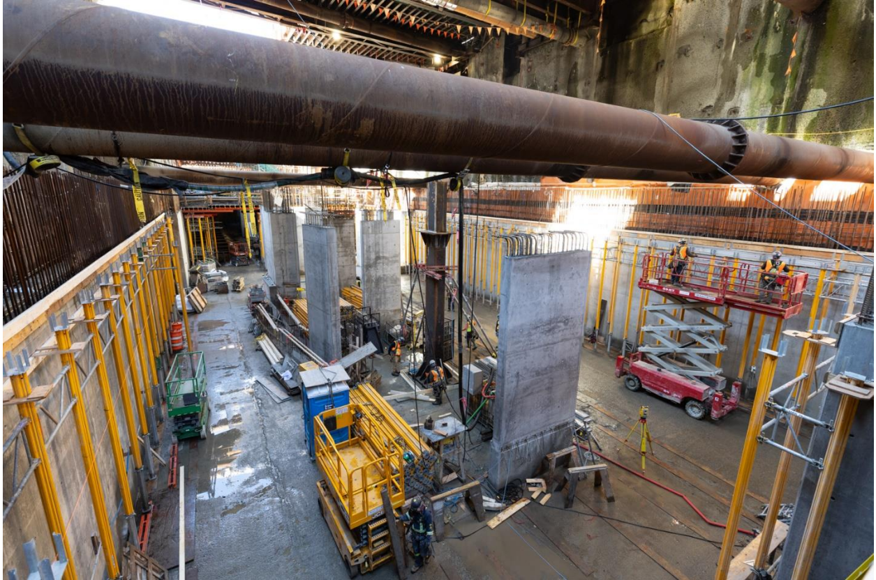
Figure 4: Broadway-City Hall Station: Progressing with shoring installation to construct the concourse level in the station box.
