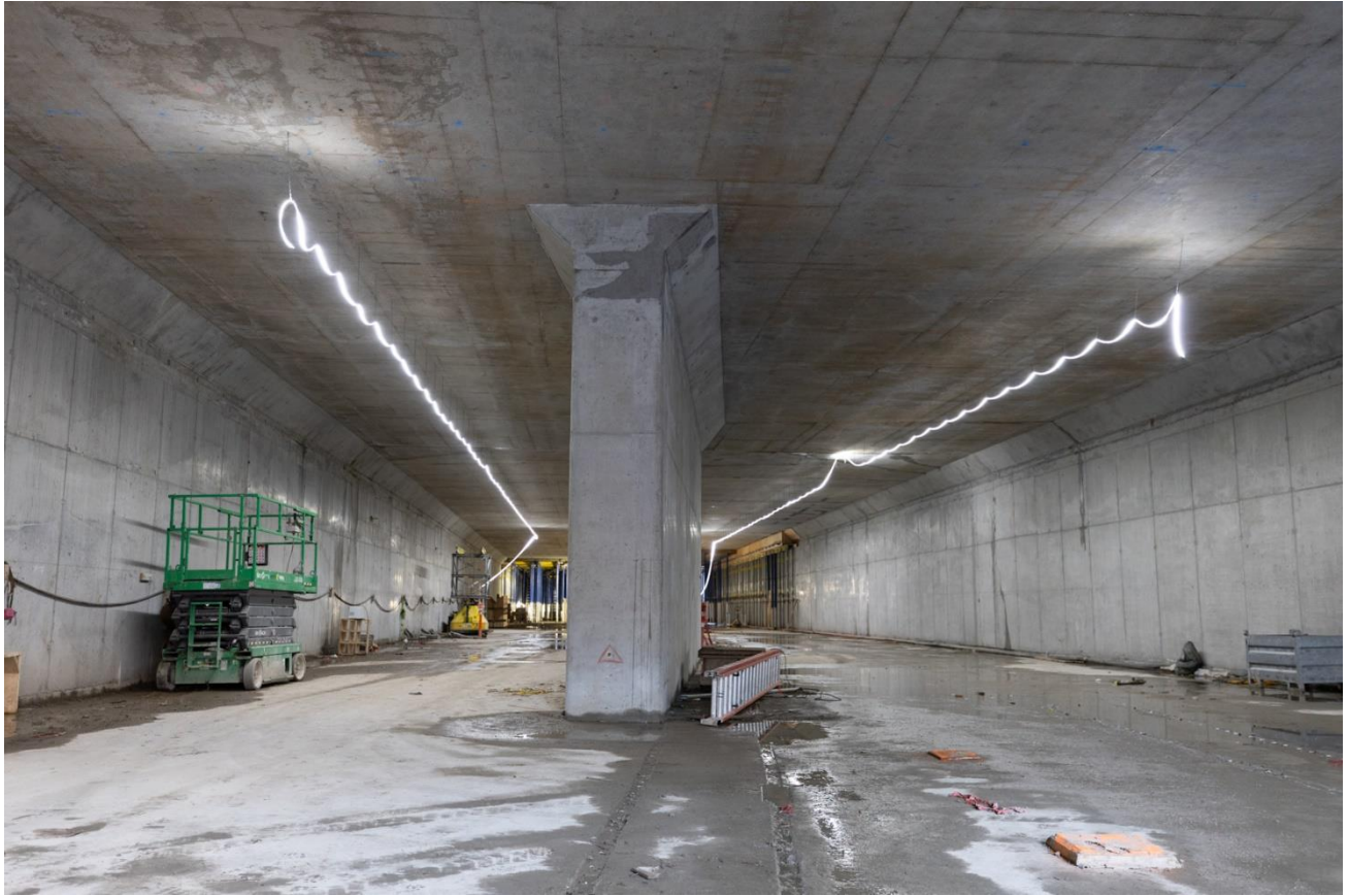
Figure 7: Arbutus Station: Progressing with construction of the crossover box roof.
