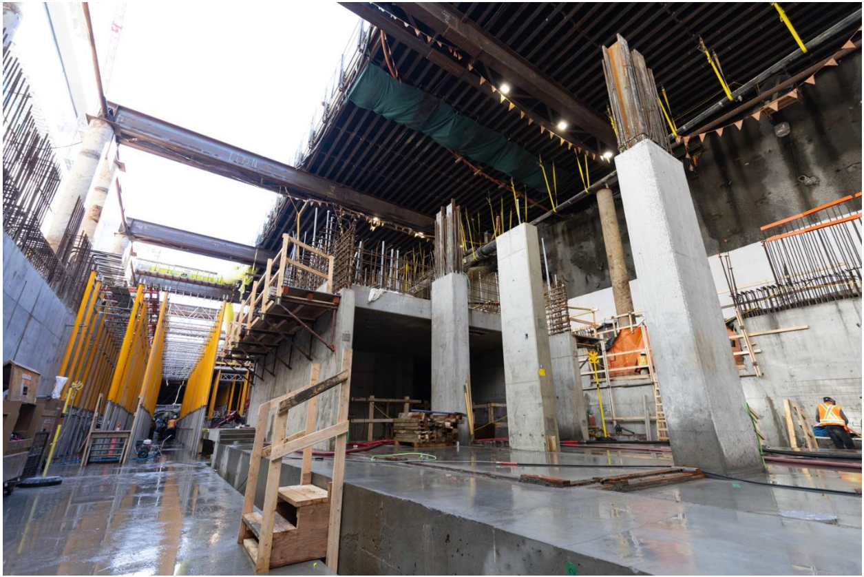
Figure 6: South Granville Station: Progressing with construction of the concourse level floor in the station box.
