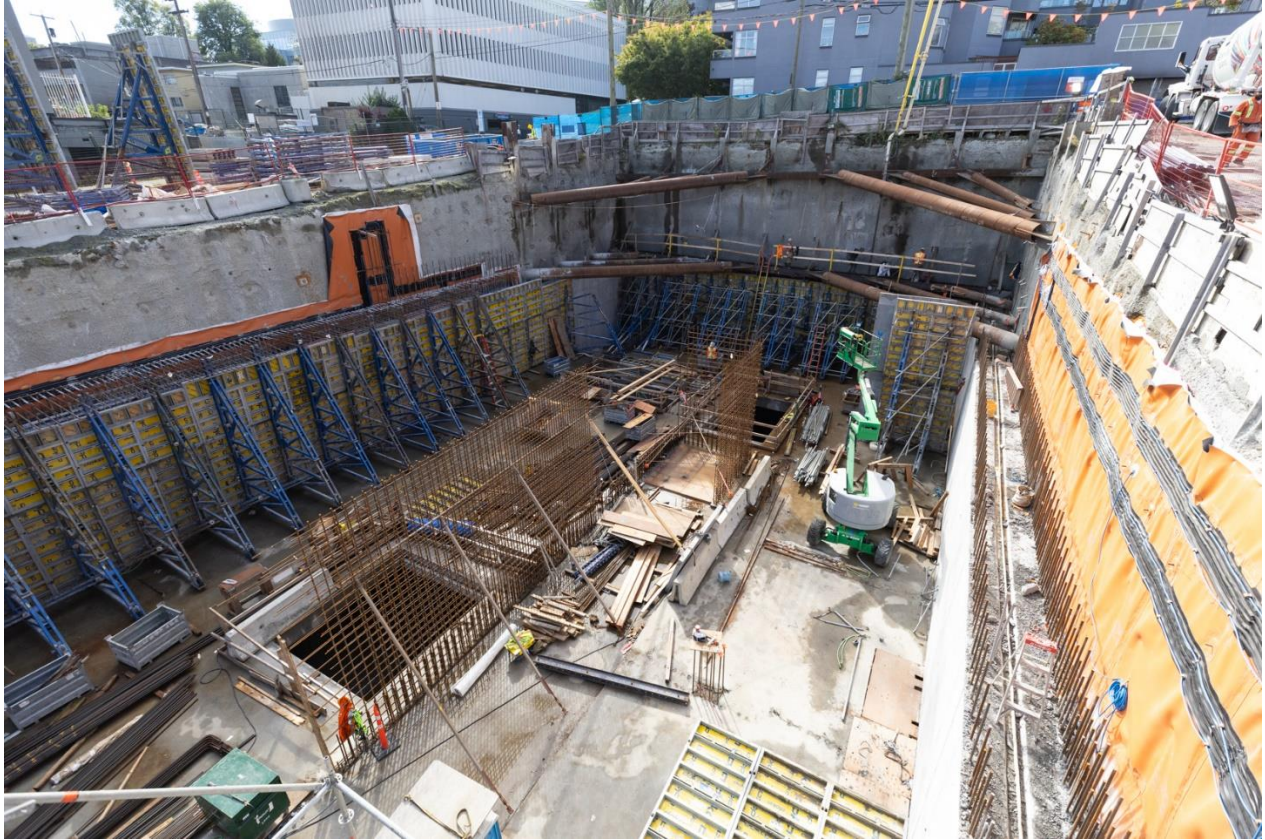
Figure 5: Oak-VGH Station: Progressing with rebar installation and concrete pours for the concourse-level walls in the headhouse.
