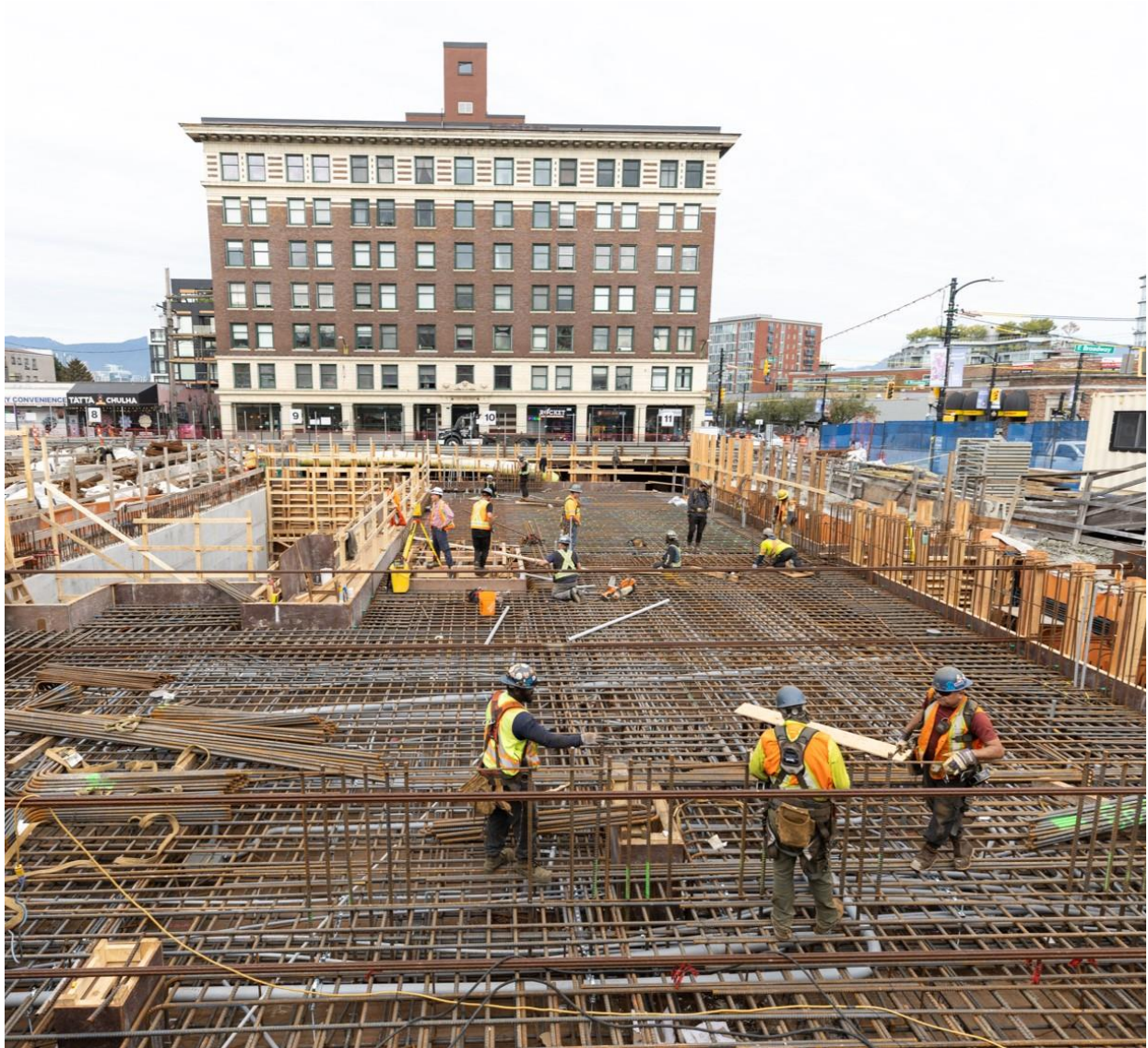
Figure 3: Mount Pleasant Station: Progressing with rebar installation for the roof slab in the headhouse.
