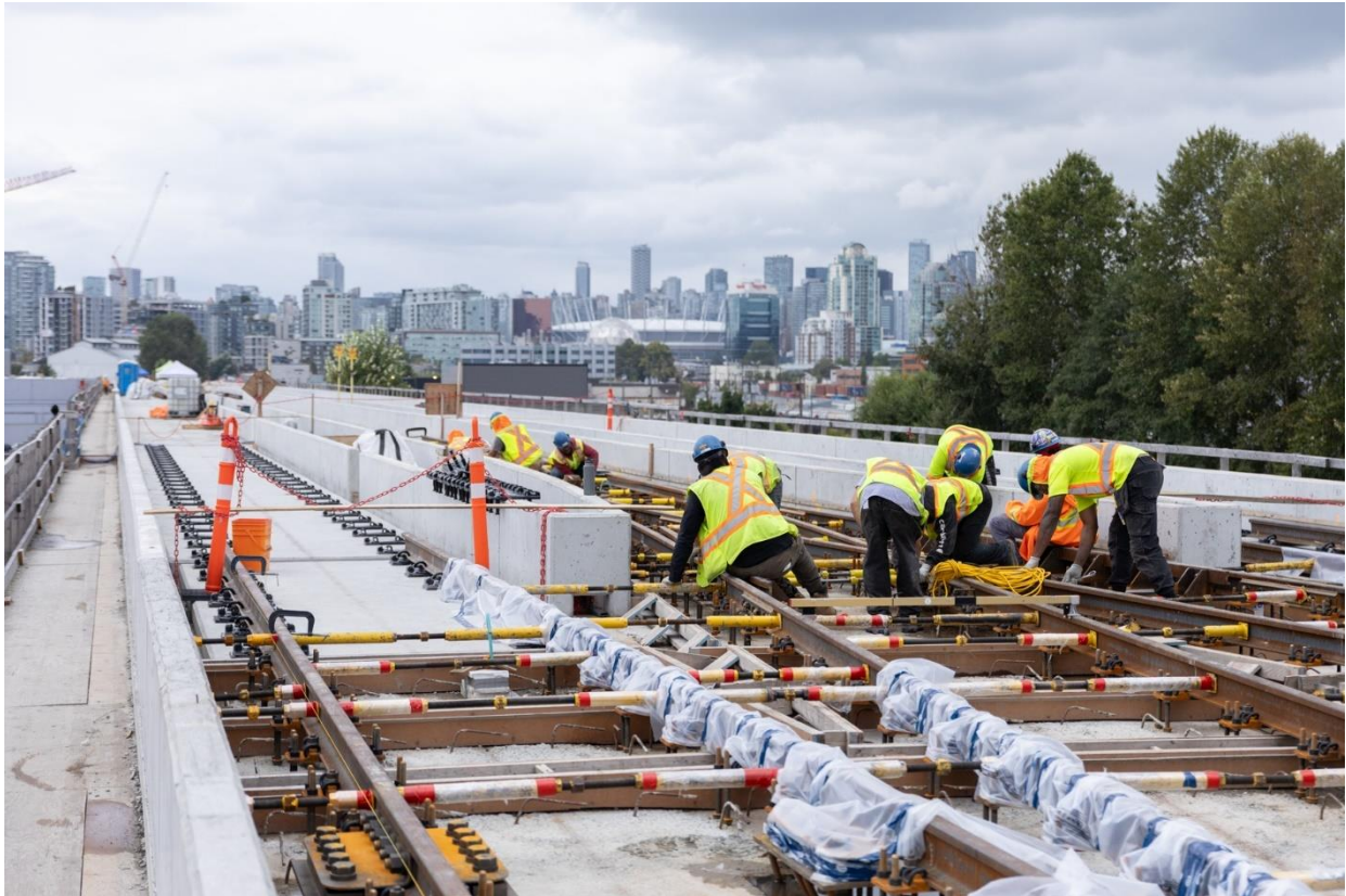
Figure 1: Elevated Guideway: Progressing with aligning the track switches for the pocket track.
