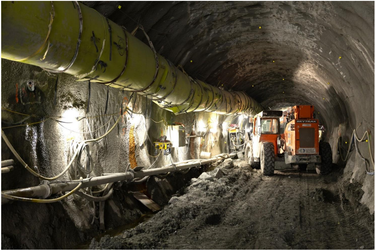
Figure 7: Arbutus Station: Progressing with excavation of the tail track tunnels west of the station box.
