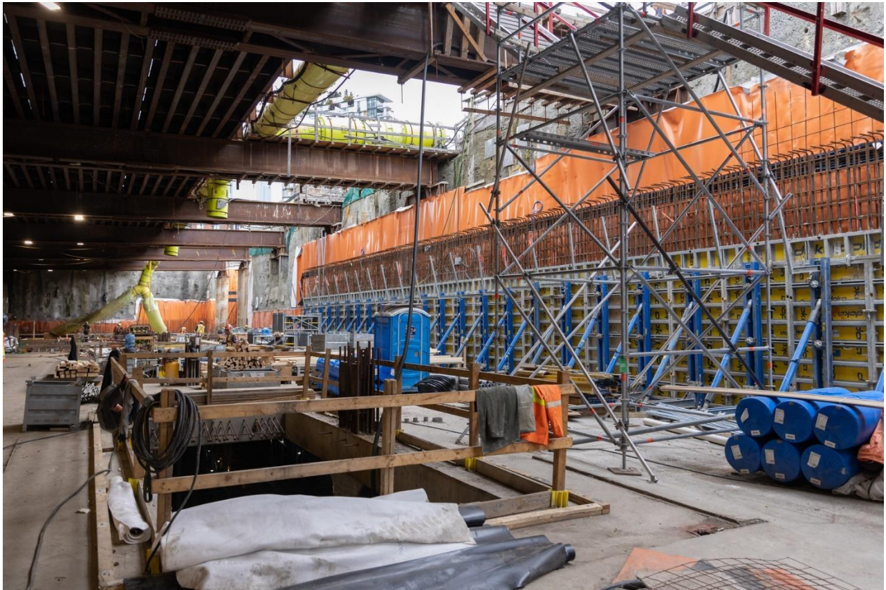
Figure 3: Mount Pleasant Station: Progressing with the concourse-level walls in the station box.
