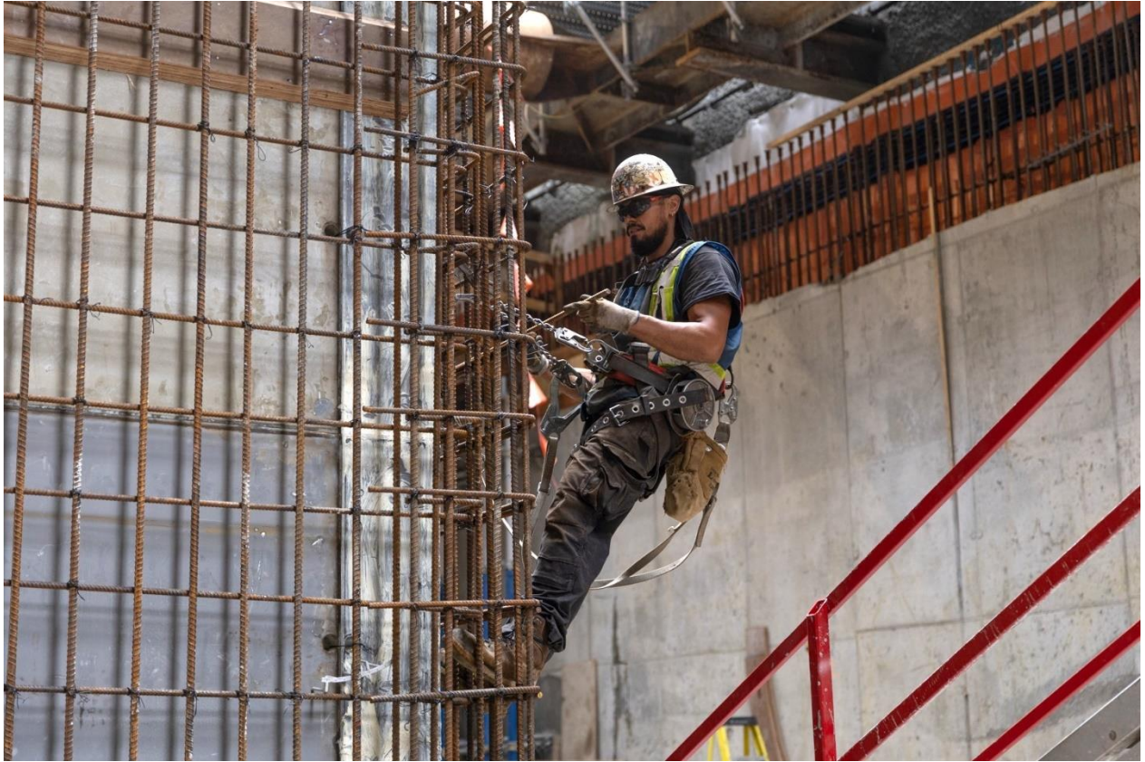
Figure 5: Oak-VGH Station: Progressing with rebar installation for the columns in the station box.
