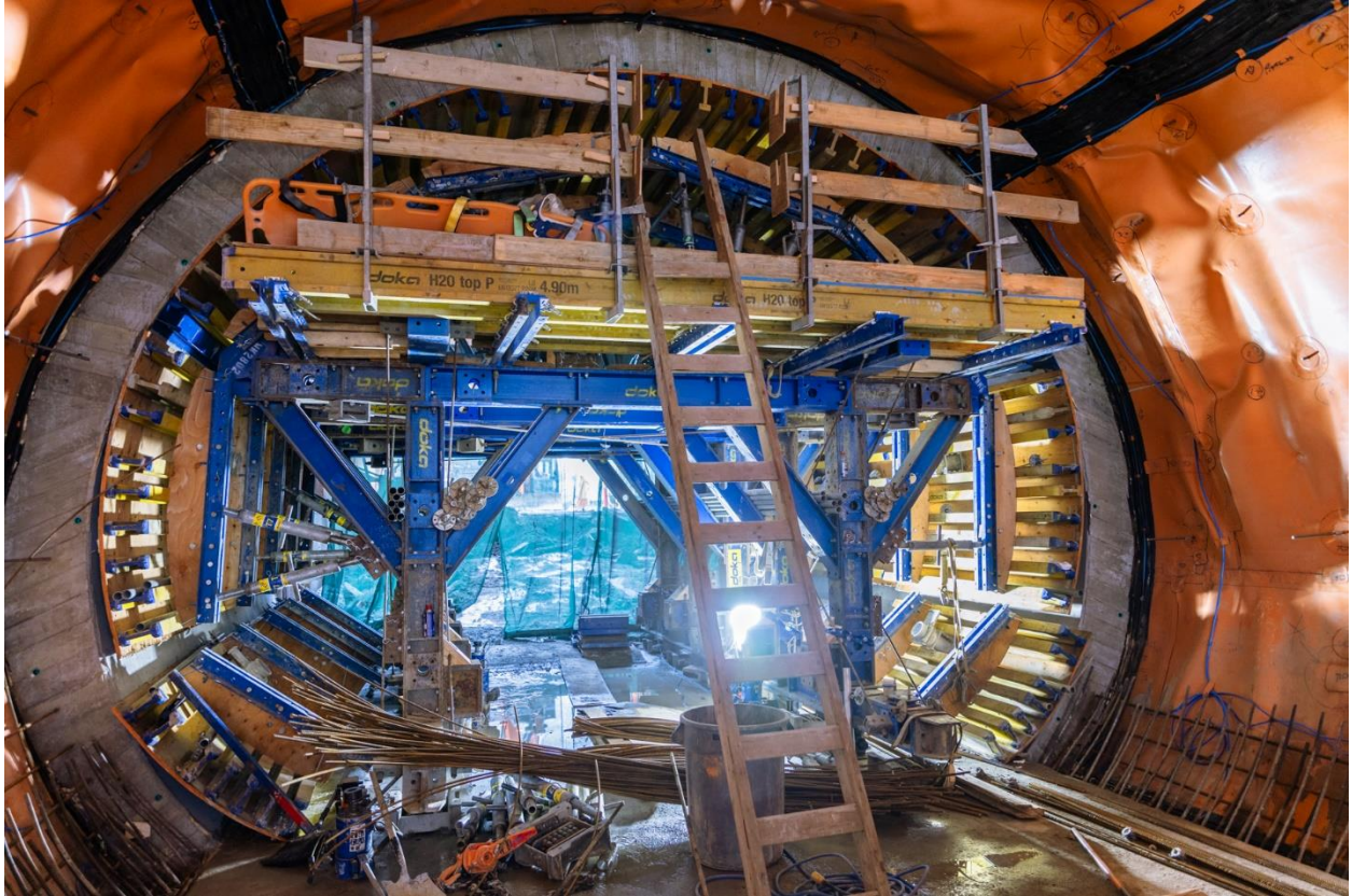
Figure 4: Broadway-City Hall Station: Progressing with concrete works to construct the tunnelled passenger connections to the Canada Line platforms.
