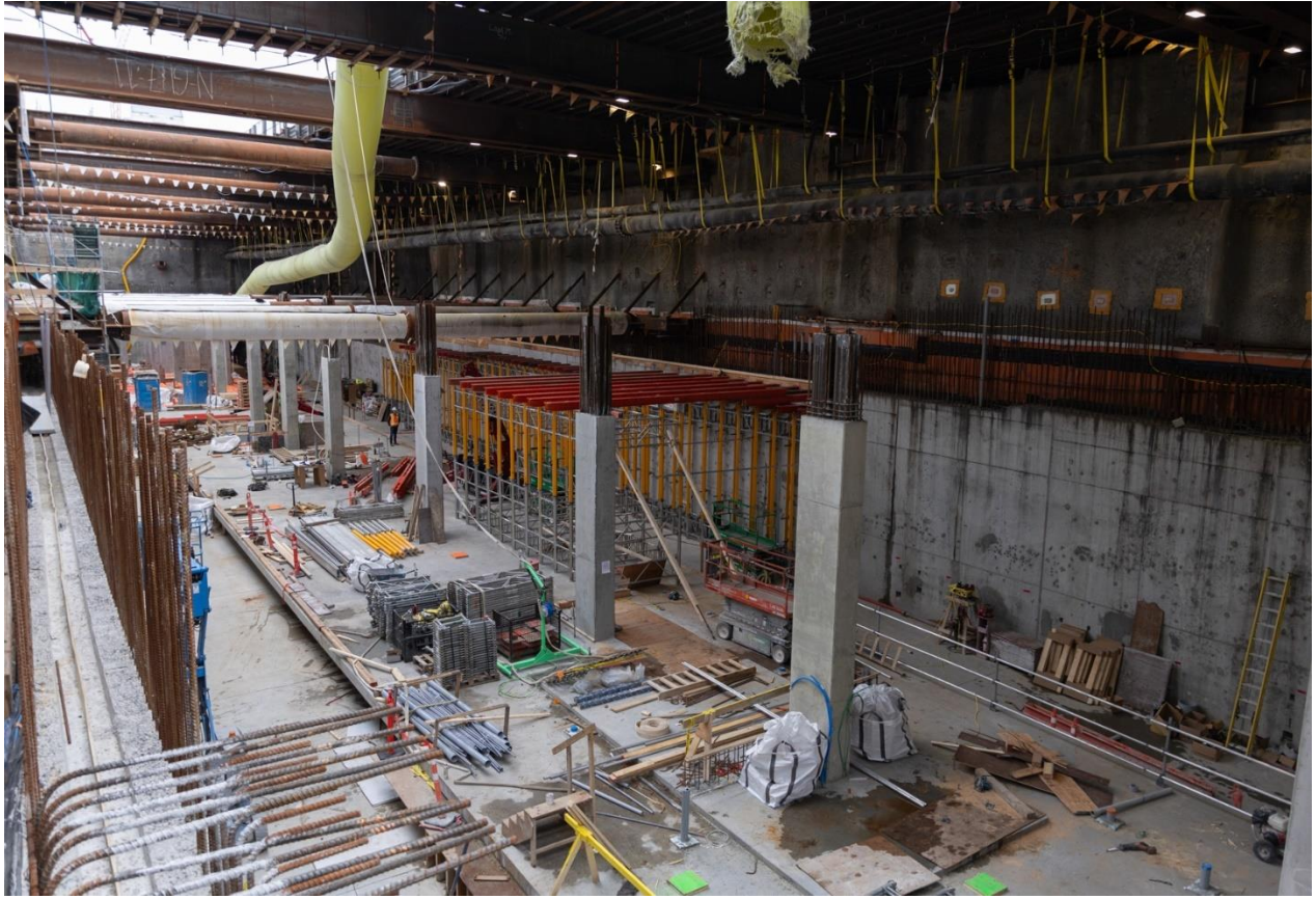
Figure 6: South Granville Station: Completion of the platform slab in the station box.
