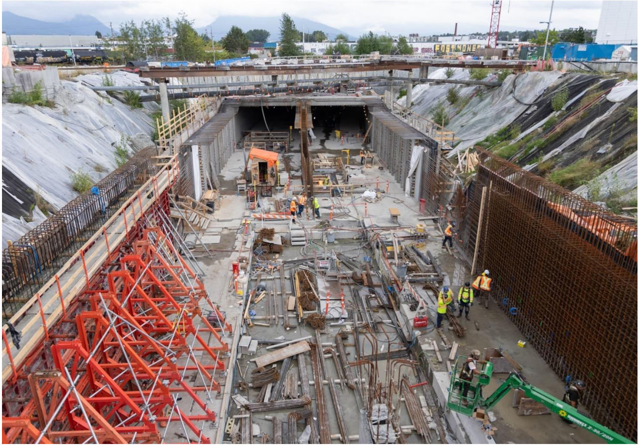
Figure 2: Great Northern Way-Emily Carr Station: Progressing with walls for the station box (shown in the foreground) and transition box (shown in the background).
