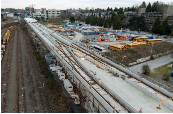
Figure 1: Elevated Guideway: Progressing with track installation.
