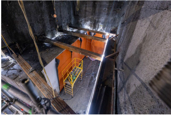
Figure 5: Oak-VGH Station: Progressing with waterproofing in the ventilation shaft.
