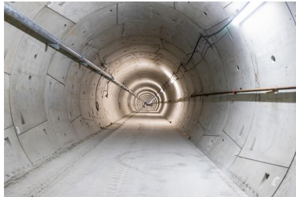
Figure 8: Tunnels: Completion of the track slab in the tunnels.
