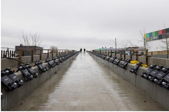
Figure 1: Elevated Guideway: Preparing to install fasteners.
