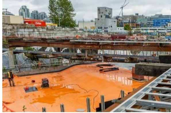
Figure 2: Great Northern Way-Emily Carr Station: Progressing with waterproofing the roof of the transition box.
