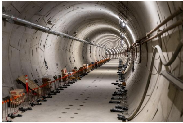
Figure 8: Tunnels: Progressing with coring in the track slab for the installation of track fasteners in the outbound tunnel.
