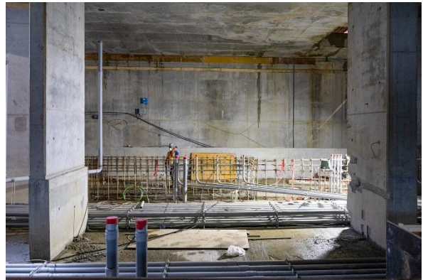
Figure 4: Broadway-City Hall Station: Progressing with rebar and conduit installation for the station platform.
