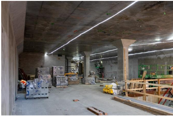
Figure 7: Arbutus Station: Progressing with construction of the masonry walls on the concourse level.
