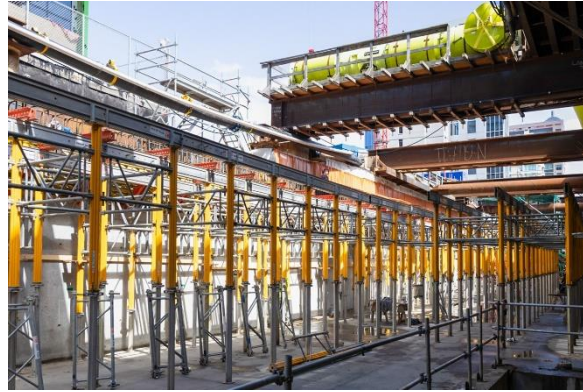
Figure 6: South Granville Station: Progressing with installation of shoring for the roof slab.
