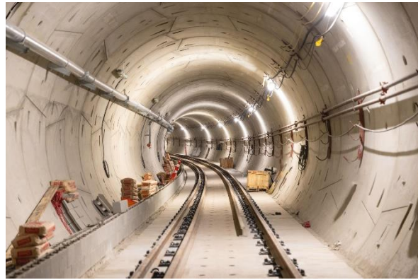
Figure 8: Tunnels: Progressing with pulling rail for track installation in the tunnels between Great Northern Way-Emily Carr and Broadway-City Hall stations.
