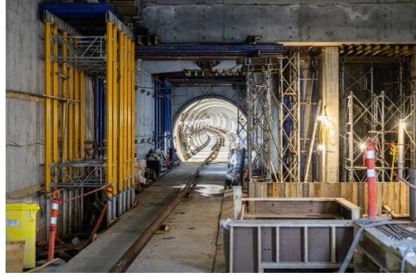
Figure 2: Great Northern Way-Emily Carr Station: Progressing with pulling rail through the station and into the tunnels.
