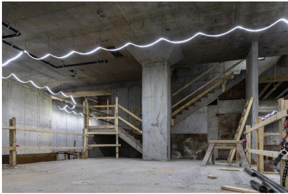
Figure 7: Arbutus Station: Progressing with construction of the emergency exit stairs at the east end of the platform.
