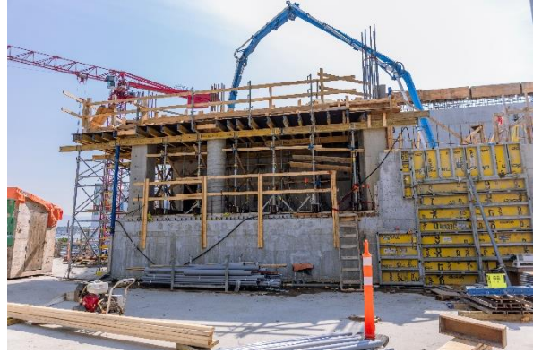
Figure 2: Great Northern Way-Emily Carr Station: Progressing with concrete pours to construct the above-ground station entrance.
