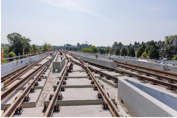
Figure 1: Elevated Guideway: Progressing with rail pulling and installation.
