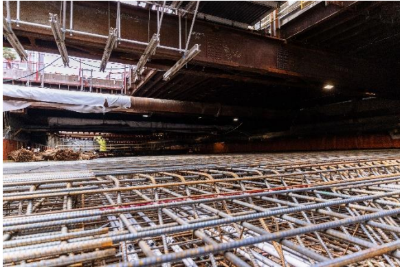
Figure 5: Oak-VGH Station: Progressing with construction of the roof of the station box.
