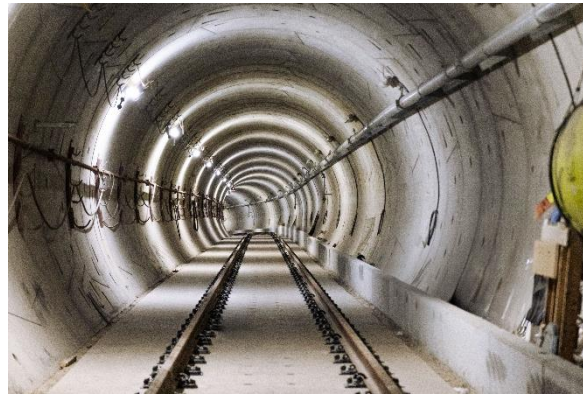
Figure 8: Tunnels: Progressing with pulling rail for track installation in the tunnels.
