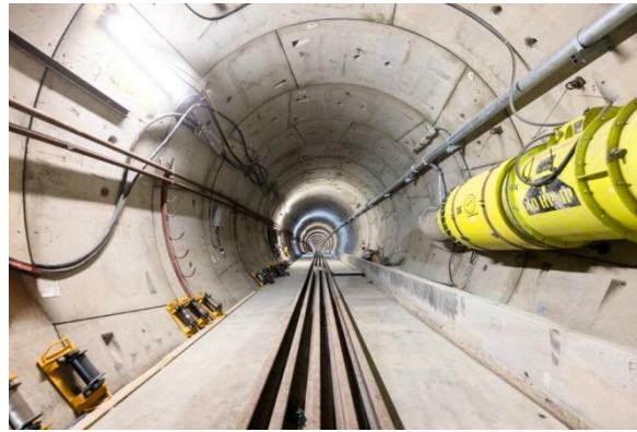
Figure 8: Tunnels: Progressing with pulling rail for track installation in the tunnels between Broadway-City Hall and Oak-VGH stations.
