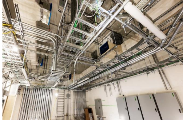
Figure 2: Great Northern Way-Emily Carr Station: Progressing with installation of mechanical, electrical, and plumbing systems inside the station.
