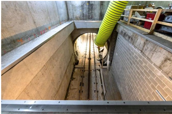
Figure 3: Mount Pleasant Station: Preparing to install tunnel ventilation equipment.
