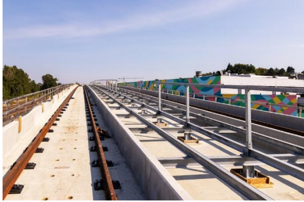
Figure 1: Elevated Guideway: Progressing with installing the walkway.
