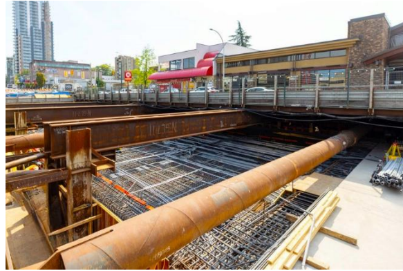
Figure 6: South Granville Station: Progressing with rebar installation for the roof slab.
