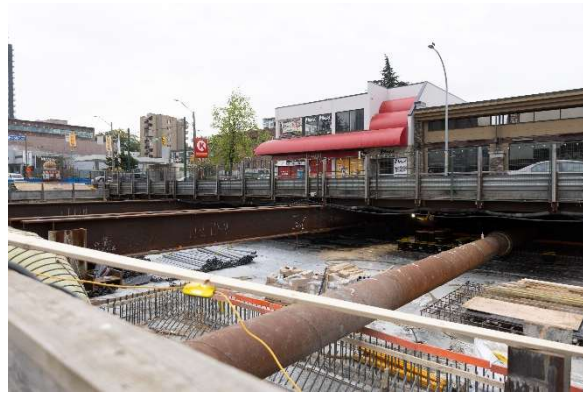
Figure 6: South Granville Station: Progressing with construction of the station box roof slab.
