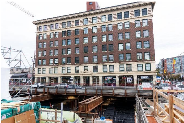
Figure 3: Mount Pleasant Station: Progressing with waterproofing on the station box roof.
