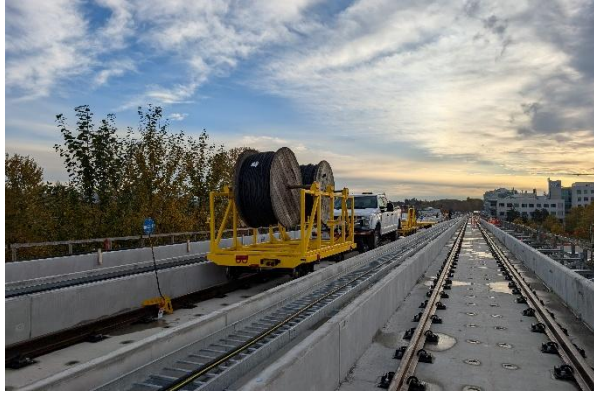
Figure 1: Elevated Guideway: Progressing with cable pulling for systems.
