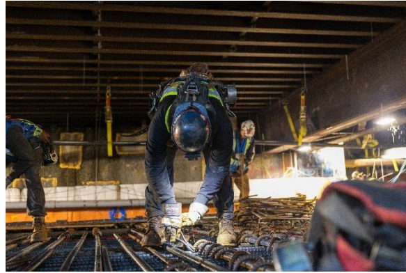
Figure 6: South Granville Station: Progressing with rebar installation for the final segment of the underground station roof.
