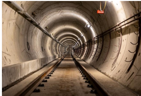
Figure 8: Tunnels: Progressing with alignment and installation of running rail west of Broadway-City Hall Station.
