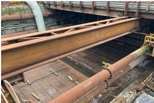
Figure 7: Arbutus Station: Progressing with rebar installation for the roof in the crossover section.
