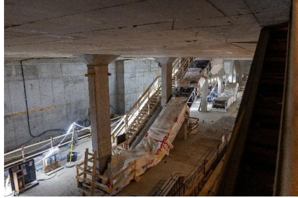
Figure 2: Great Northern Way-Emily Carr Station: Progressing with installation of escalators at the platform level.
