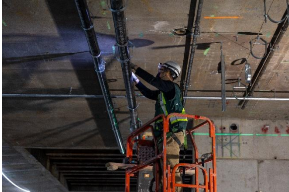
Figure 5: Oak-VGH Station: Progressing with installation of mechanical, electrical and plumbing systems in the station.
