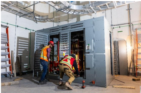
Figure 3: Mount Pleasant Station: Progressing with installation of propulsion power substation equipment.
