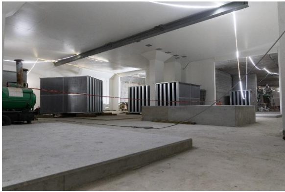
Figure 5: Oak-VGH Station: Progressing with station fit-out of the tunnel ventilation system.
