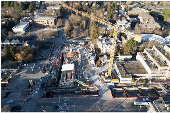
Figure 7: Arbutus Station: Progressing with waterproofing the underground station roof.
