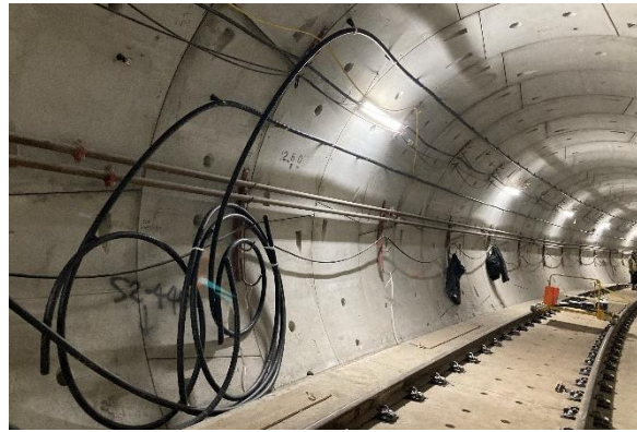
Figure 8: Tunnels: Progressing with pulling cables through the tunnels for systems.
