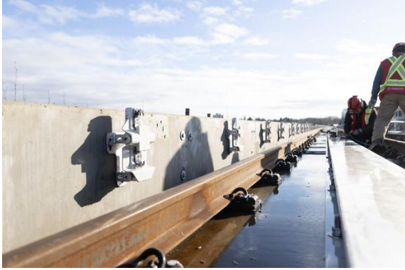
Figure 1: Elevated Guideway: Progressing with installing the power rail.
