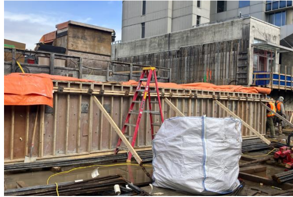
Figure 6: South Granville Station: Progressing with construction of the ventilation shafts.
