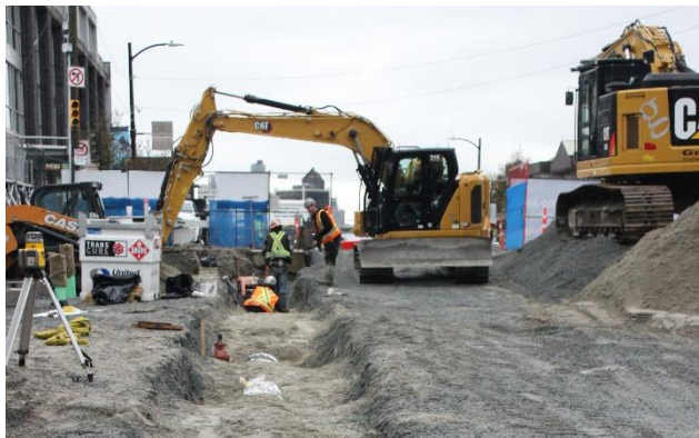
Figure 3: Mount Pleasant Station: Progressing with permanent utility relocation on E. Broadway.
