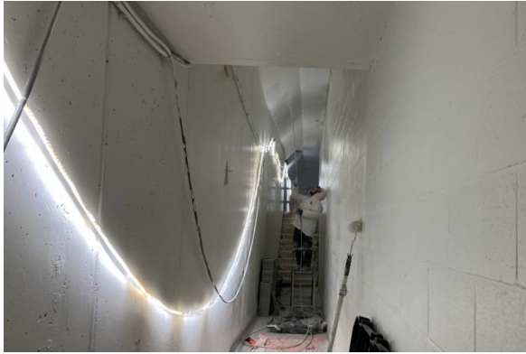
Figure 5: Oak-VGH Station: Progressing with station fit-out.
