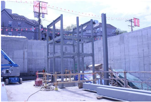
Figure 5: Oak-VGH Station: Progressing with installation of the above-ground steel structure.
