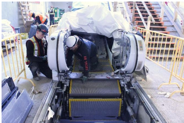
Figure 7: Arbutus Station: Progressing with installation of the escalators.
