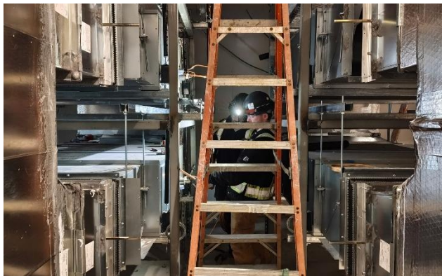
Figure 3: Mount Pleasant Station: Progressing with fit-out of the air conditioning systems.
