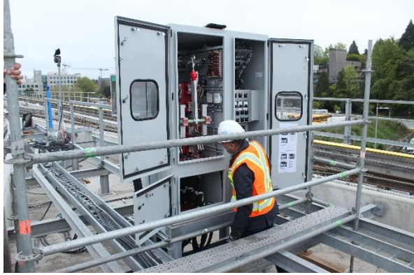
Figure 1: Elevated Guideway: Progressing with systems installation.
