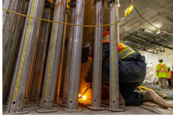
Figure 6: South Granville Station: Progressing with removal of traffic deck columns under W. Broadway.
