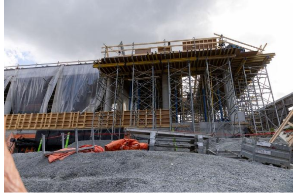
Figure 2: Great Northern Way-Emily Carr Station: Completing the final concrete pour for the headhouse roof.
