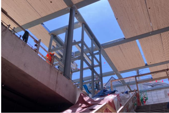
Figure 5: Oak-VGH Station: Progressing with installation of the dowel laminated timber ceiling panels for the above-ground station entrance.
