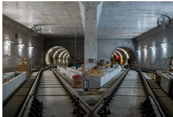
Figure 8: Tunnels: Progressing with installation of LIM and power rail in the diamond crossover east of Broadway-City Hall Station.
