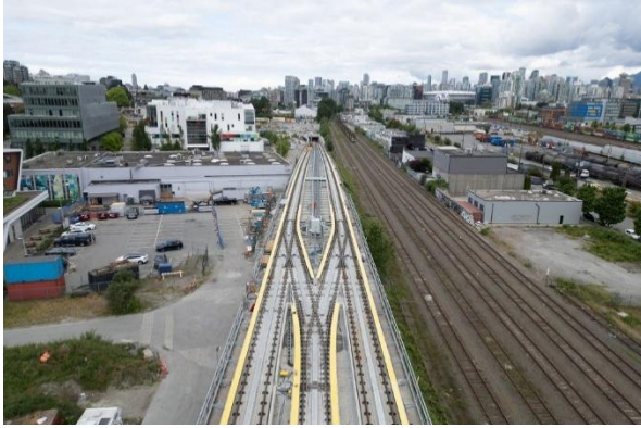
Figure 1: Elevated Guideway: Ready to begin dynamic testing.
