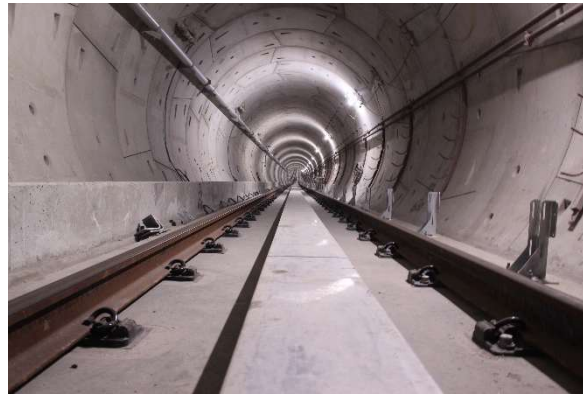
Figure 8: Tunnels: Looking west near Broadway-City Hall Station.
