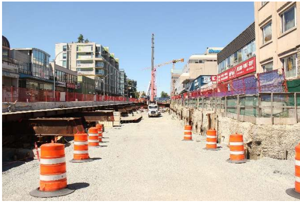
Figure 7: Arbutus Station: Progressing with removal of the traffic deck.
