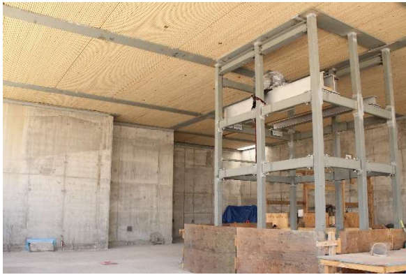
Figure 5: Oak-VGH Station: Progressing with installation of elevator structure.
