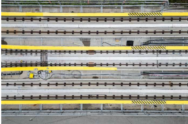
Figure 1: Elevated Guideway: Looking down on the tracks.
