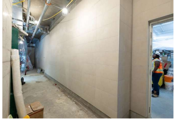
Figure 2: Mount Pleasant Station: Progressing with installation of wall tiles in the public areas of the concourse level.
