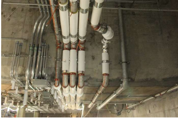
Figure 1: Great Northern Way-Emily Carr Station: Progressing with installation of mechanical, electrical, and plumbing systems at the platform level.
