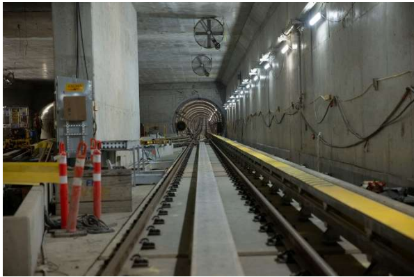
Figure 7: Tunnels: Progressing with installation of the power rail coverboards in the diamond crossover.
